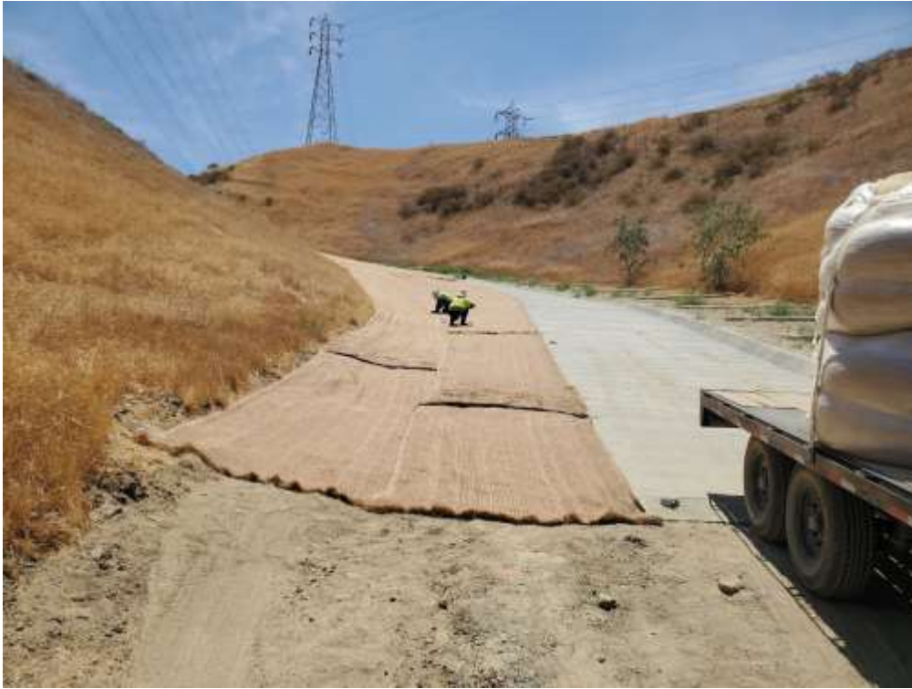
Photo 1 – BMP installation at Construction Area 2N18, Segment 2 (July 21, 2021).
