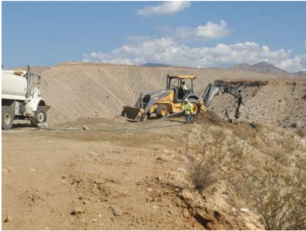
Photo 5 – Foundation wreck-out at Construction Area 6N28, Segment 6 (July 19, 2021).
