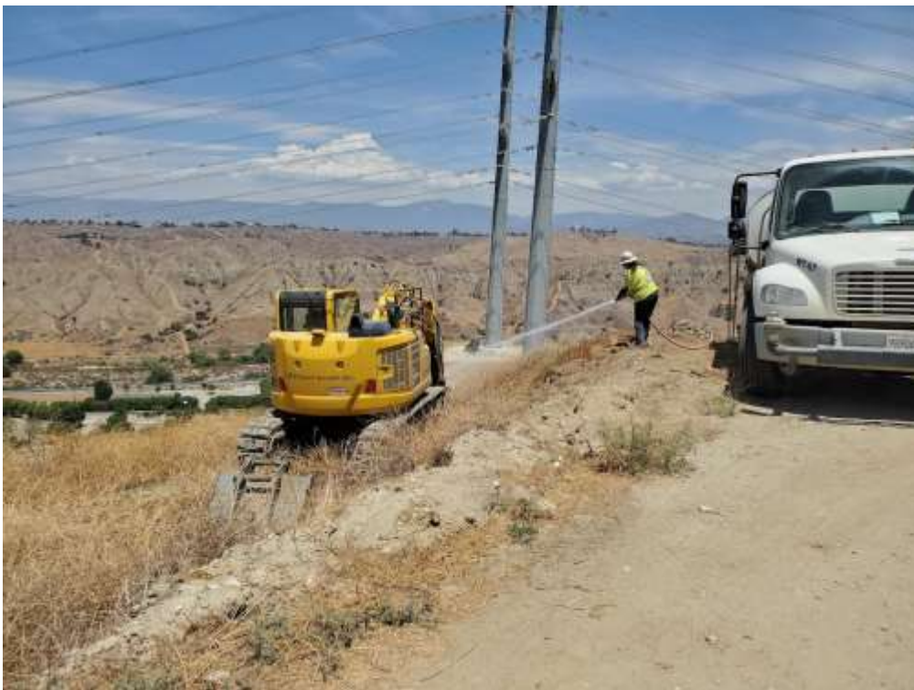
Photo 2 – Foundation wreck-out at Construction Area 3X35, Segment 3 (July 21, 2021).
