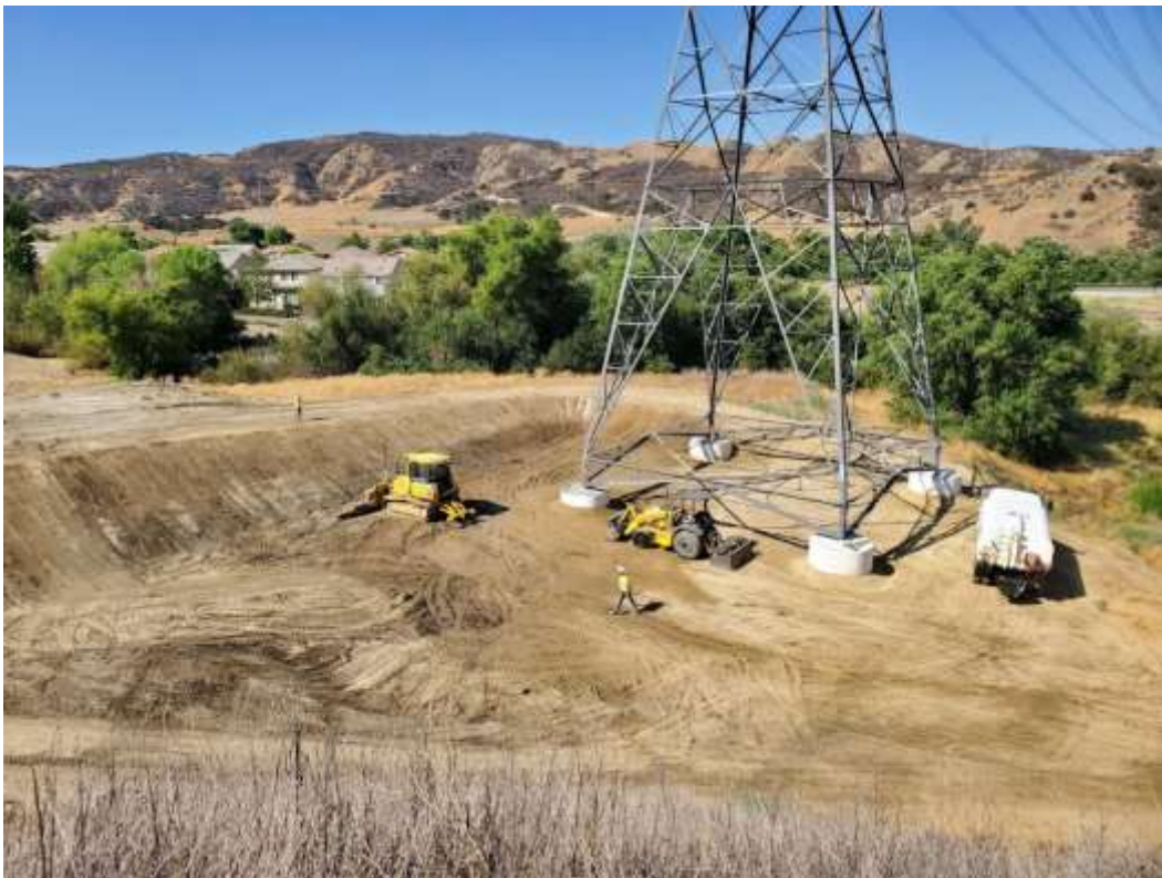
Photo 3 – Site restoration activities at Construction Area 4S60, Segment 4 (August 9, 2021).
