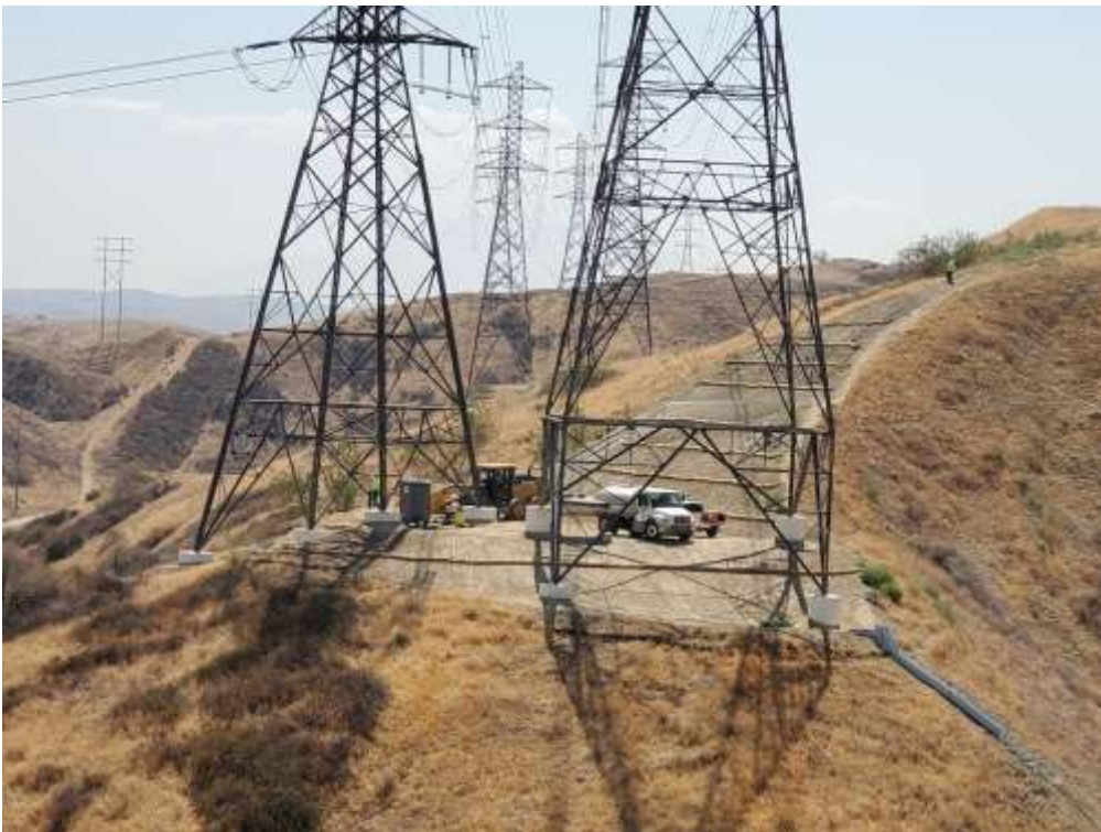
Photo 2 – Water bar installation at Construction Area 3X65, Segment 3 (August 9, 2021).
