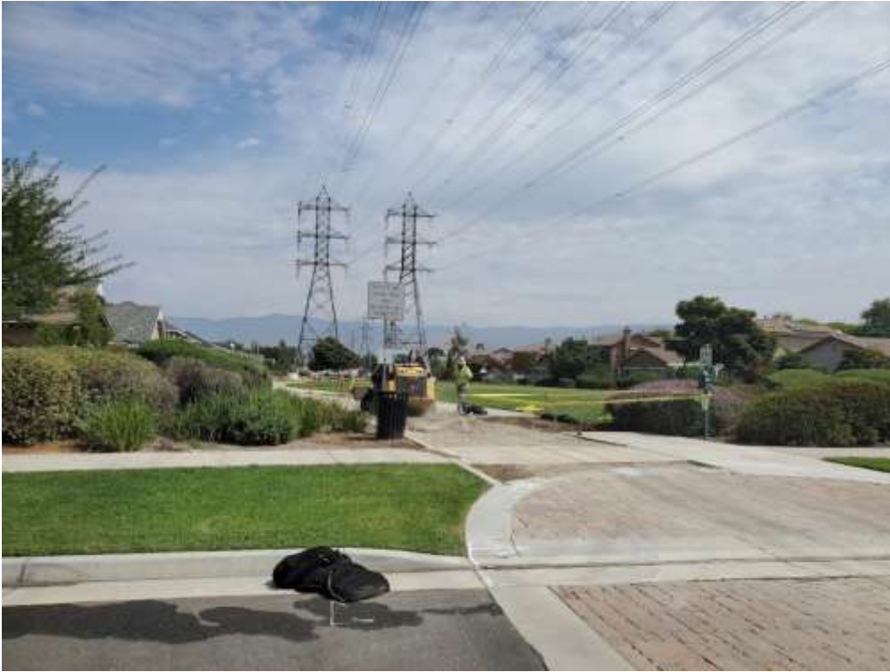
Photo 1 – Concrete replacement activities at Construction Area 1X13, Segment 1 (August 11, 2021).
