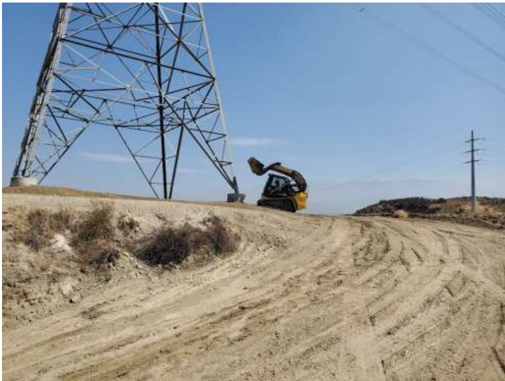
Photo 2 – Site restoration activities at Construction Area 4S58, Segment 4 (August 25, 2021).
