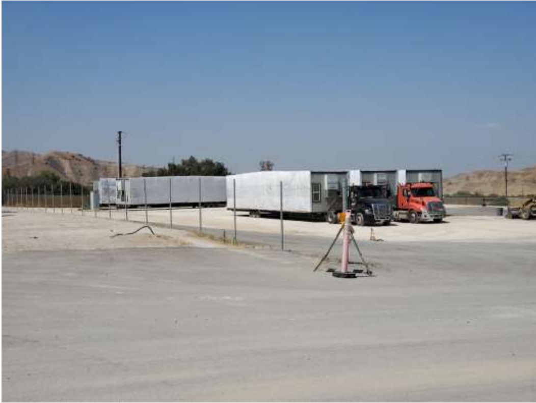
Photo 1 – Trailer demobilization at the Poultry Material Yard (September 7, 2021).
