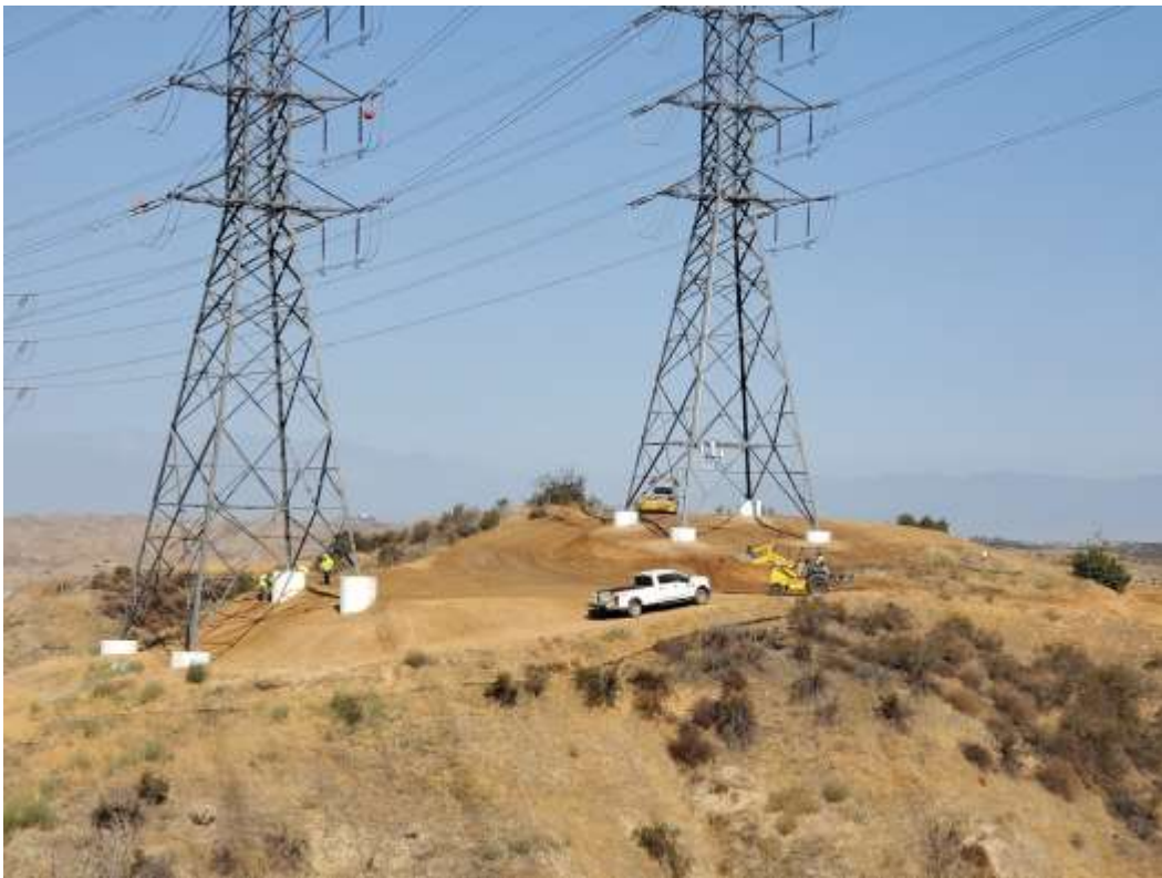
Photo 4 – Site restoration activities at Construction Area 4X57, Segment 4 (September 7, 2021).
