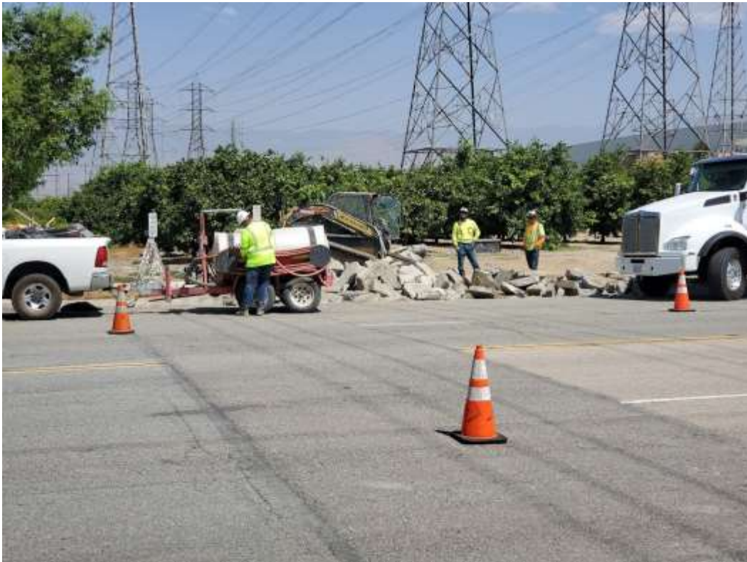
Photo 2 – Concrete repair activities at Construction Area 1X24, Segment 1 (September 7, 2021).
