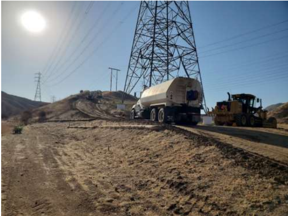
Photo 2 – Erosion repair at Construction Area 2N25, Segment 2 (September 21, 2021).
