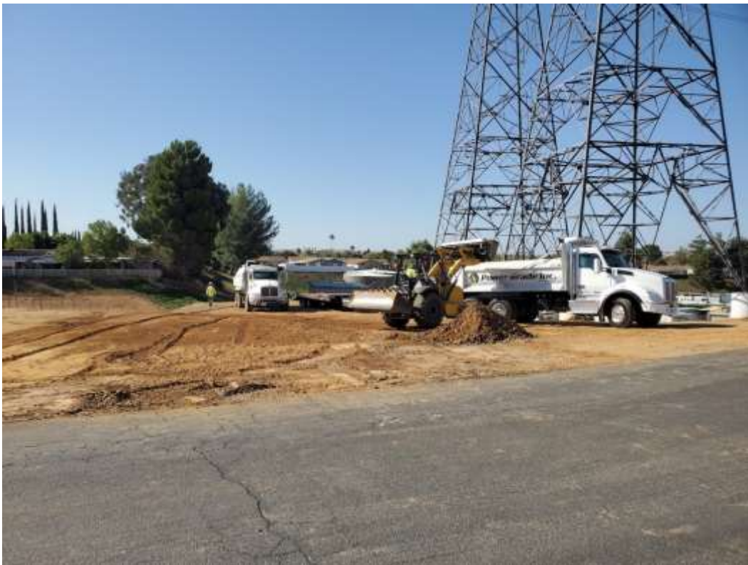
Photo 3 – Site restoration at Construction Area 4X47, Segment 4 (September 21, 2021).
