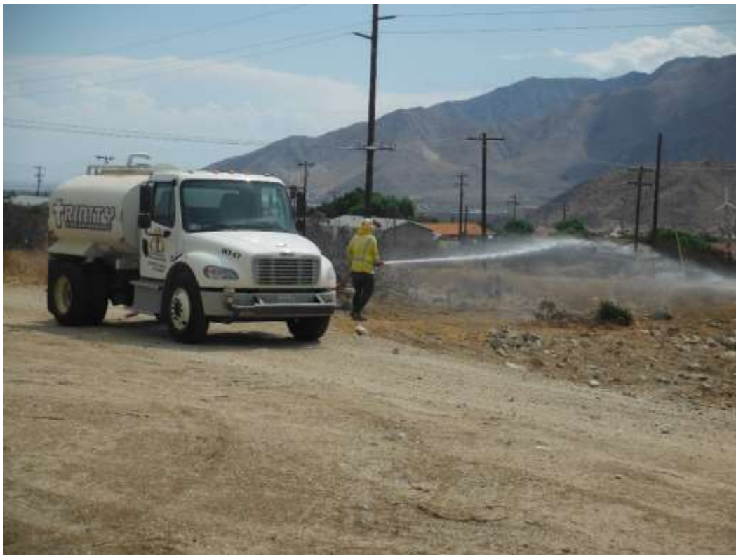
Photo 4 – Hydroseed watering at Construction Area 5X01, Segment 5 (September 23, 2021) (Photo courtesy of SCE).
