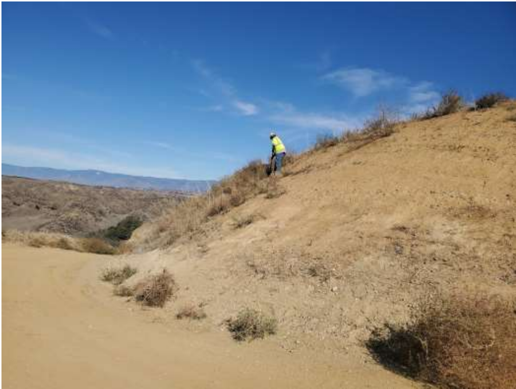
Photo 3 – Weed removal and hydroseed preparation at Construction Area 4N58, Segment 4 (November 8, 2021).
