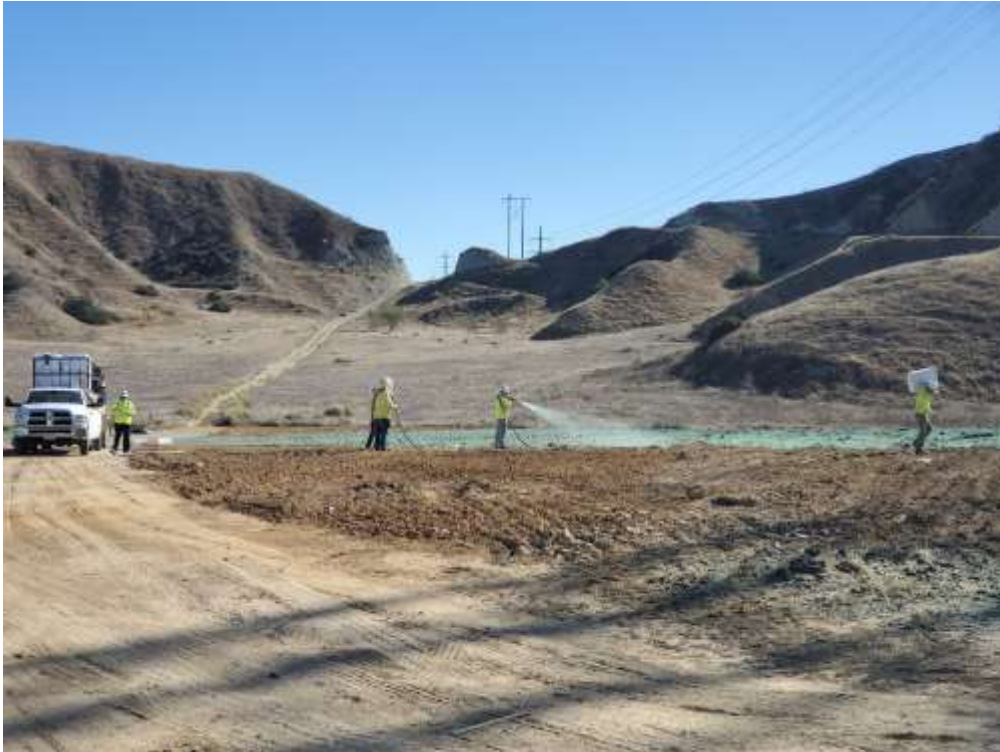
Photo 1 – Hydroseed application at Construction Area 3X06-3X07, Segment 3 (November 3, 2021).
