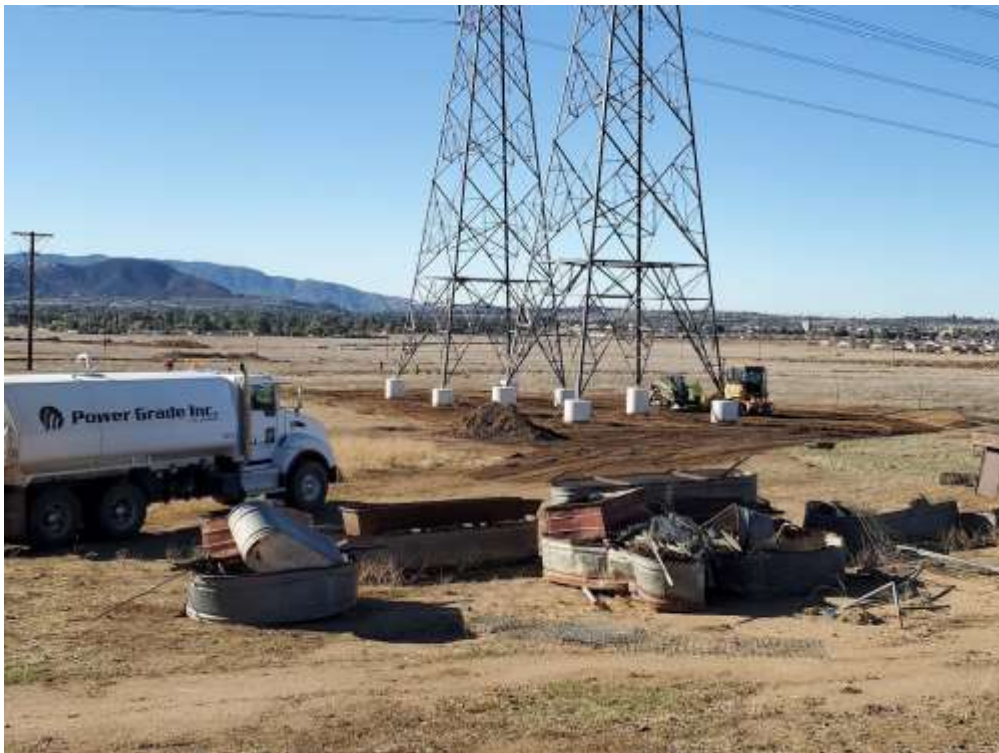
Photo 2 – Site restoration and foundation compaction at Construction Area 4X17, Segment 4 (November 3, 2021).
