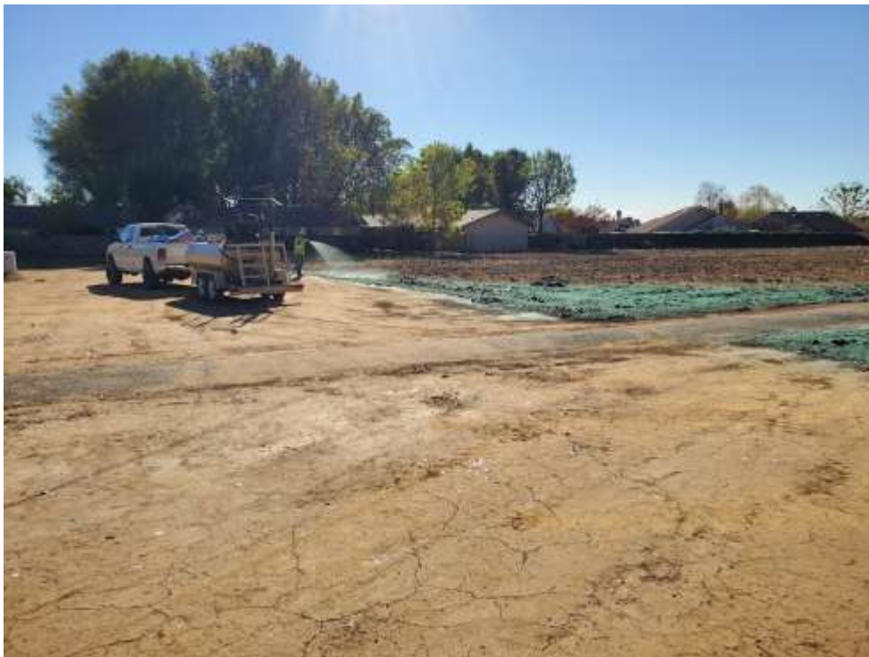
Photo 2 – Hydroseed application at Construction Area 4X29, Segment 4 (December 2, 2021).
