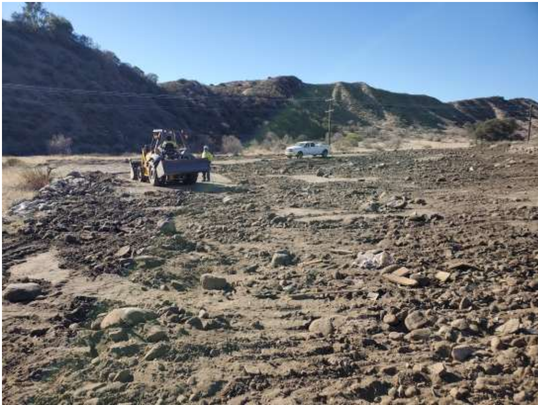
Photo 3 – Site decompaction and hydroseed preparation at Construction Area SWA-4-PP123353-4-MPR-46, Segment 4 (December 2, 2021).
