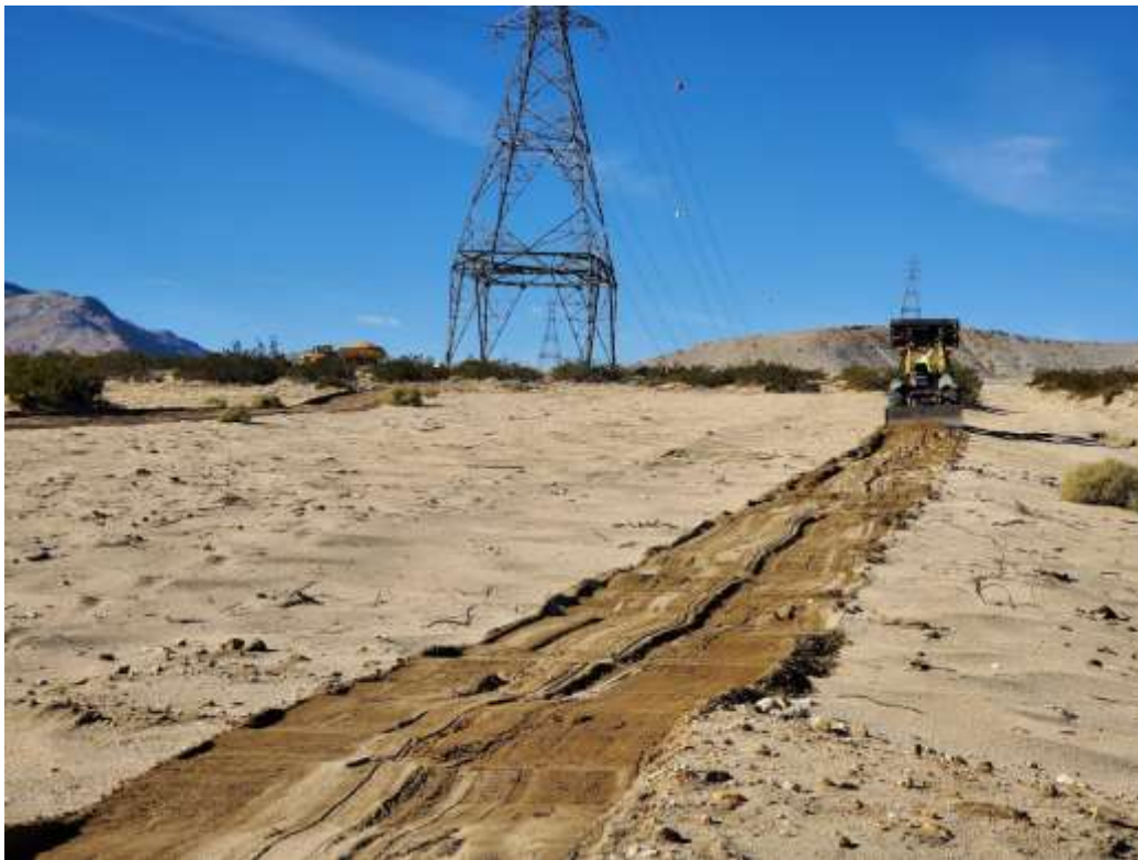
Photo 4 – Site decompaction and hydroseed preparation at Construction Area WSS-6-6N26-6N27, Segment 6 (December 20, 2021).
