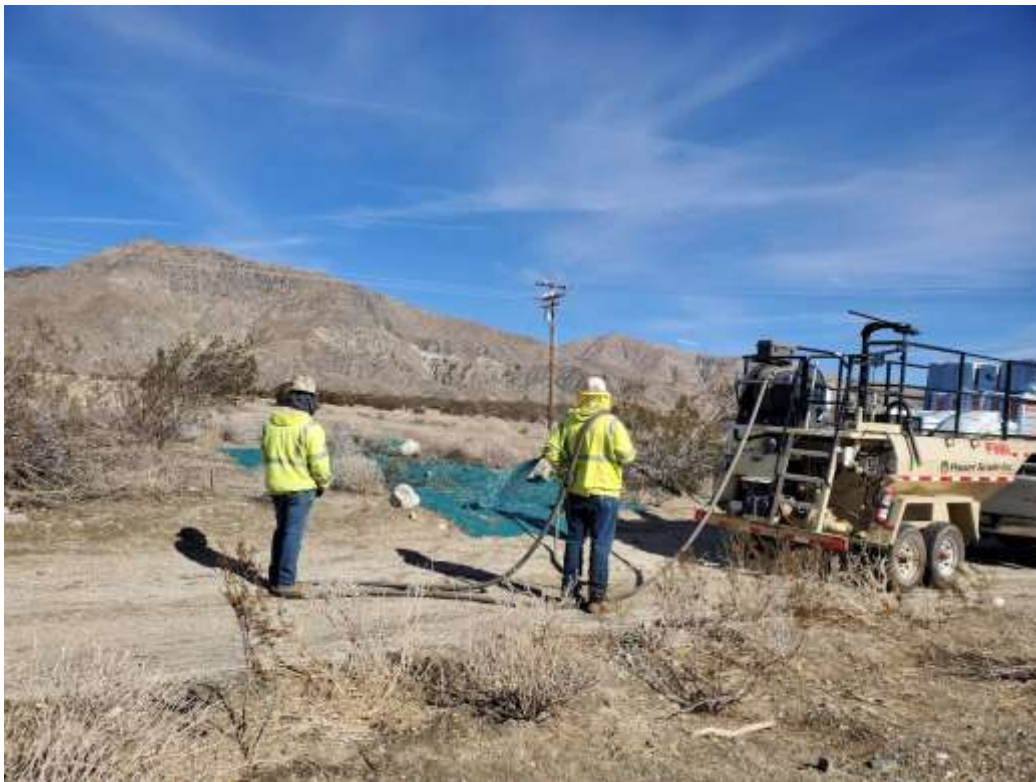
Photo 2 – Hydroseed application at Construction Area 5X01, Segment 5 (December 15, 2021).
