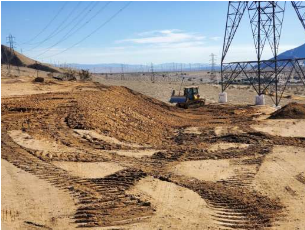
Photo 3 – Site restoration at Construction Area 6N35, Segment 6 (December 20, 2021).
