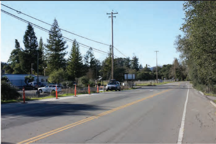
1. Old Redwood Highway near Highway 101 offramp looking north
