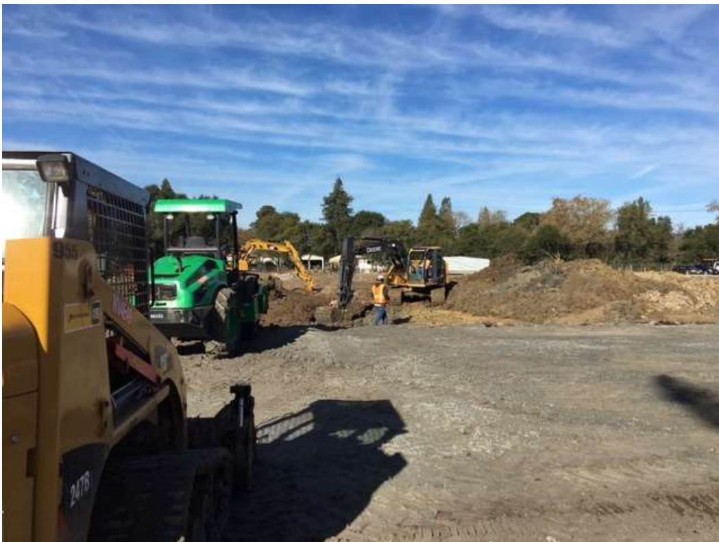
Figure 2 – Excavating from the central area of the substation site, December 20, 2016.
