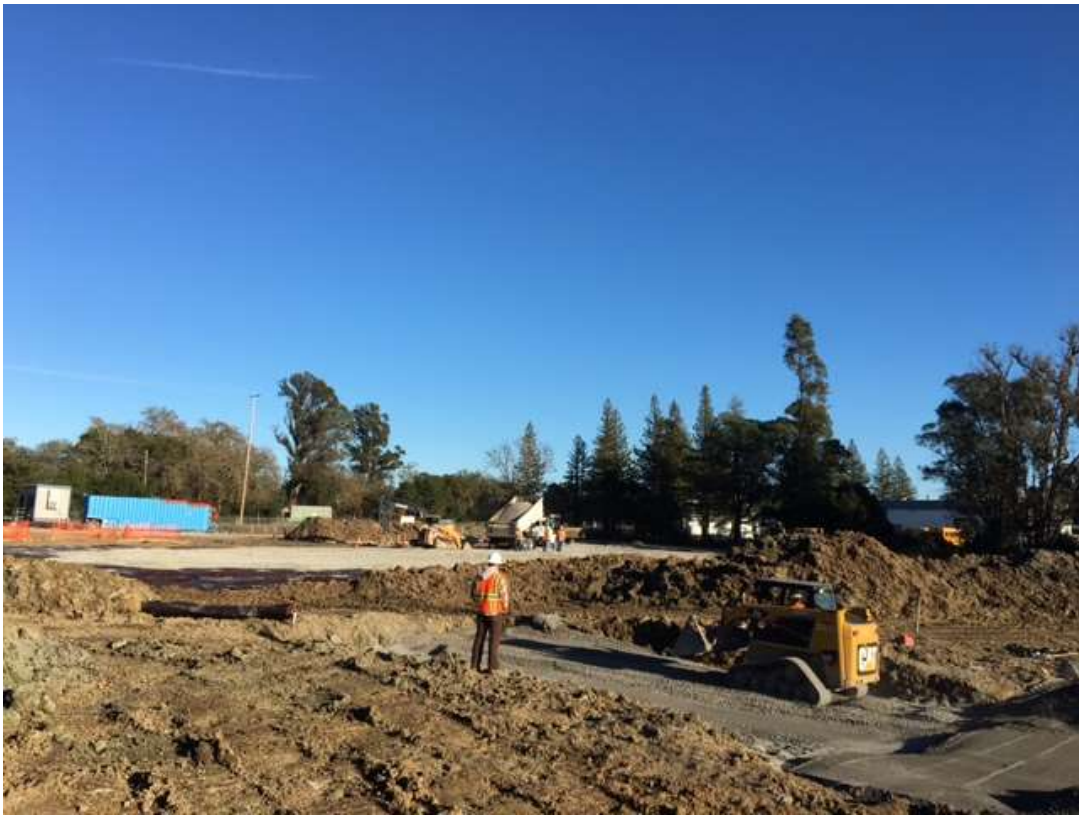
Figure 3 – Rock being delivered and compacted at the substation site, December 22, 2016.
