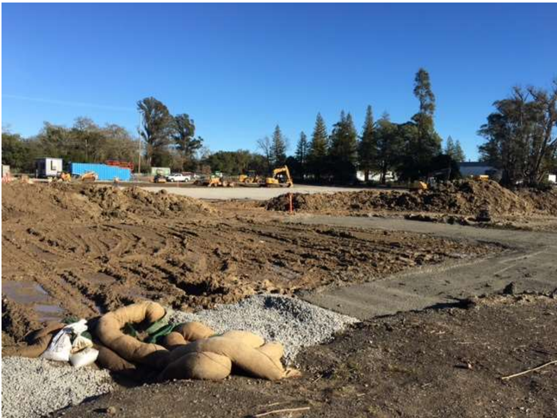
Figure 6 – Rock was delivered to substation site and compacted, December 28, 2016.
