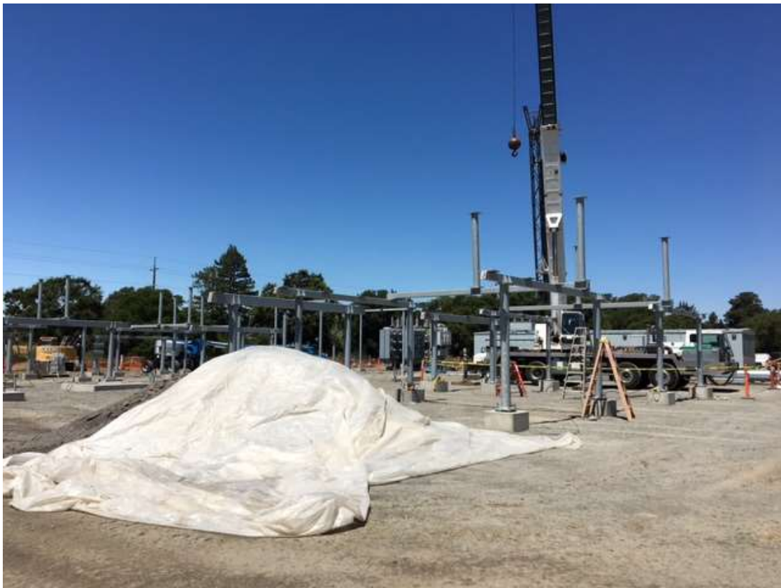
Figure 5 – Erecting steel bus structures – view northwest, July 26, 2017.
