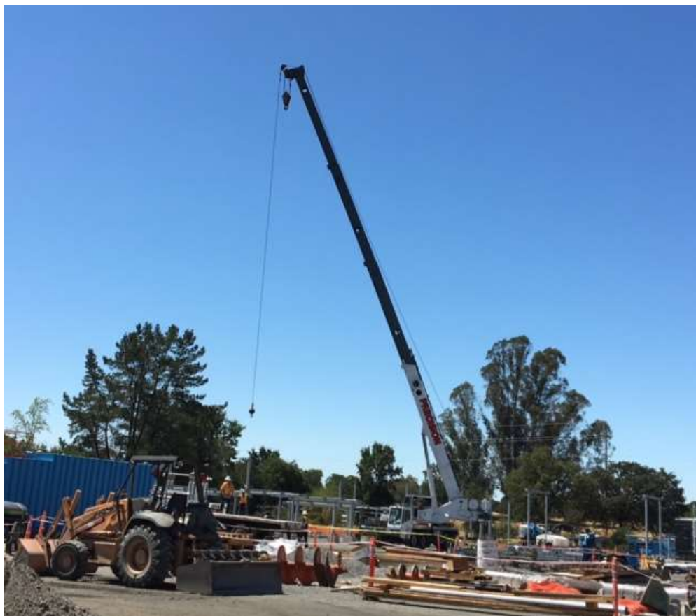
Figure 4 – Erecting steel bus structures with crane – view southwest, July 26, 2017.
