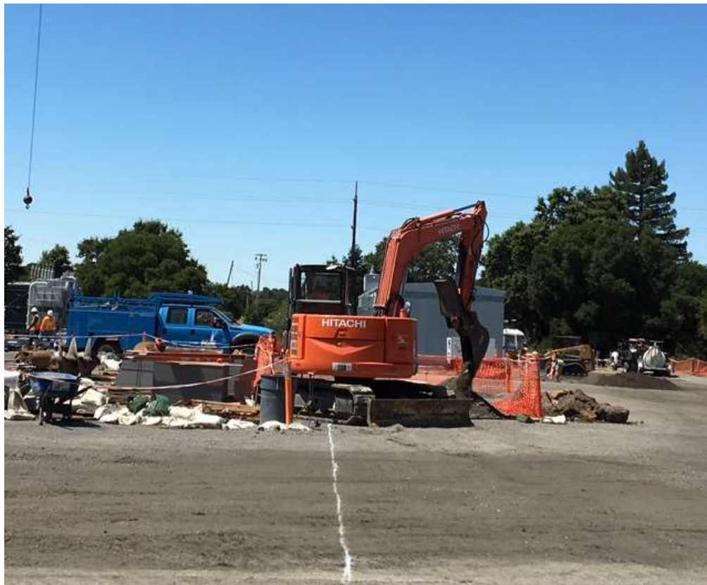
Figure 3 – Excavating for telecom line – view west, July 26, 2017.
