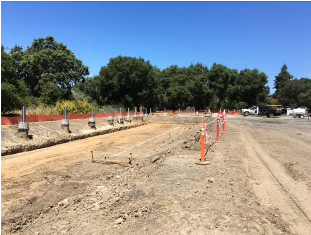
Figure 2 – SPCC pond excavation on west side of site – view north, July 26, 2017.
