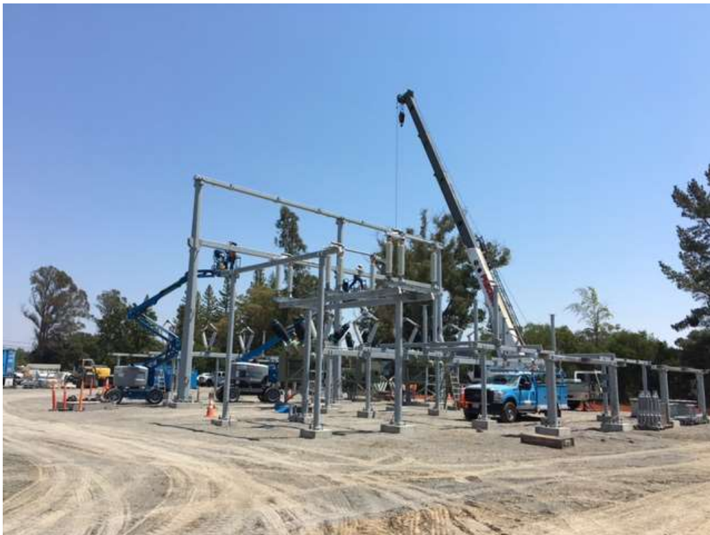
Figure 2 – Preparing to install switches on dead-end structures – view southeast, August 1, 2017.
