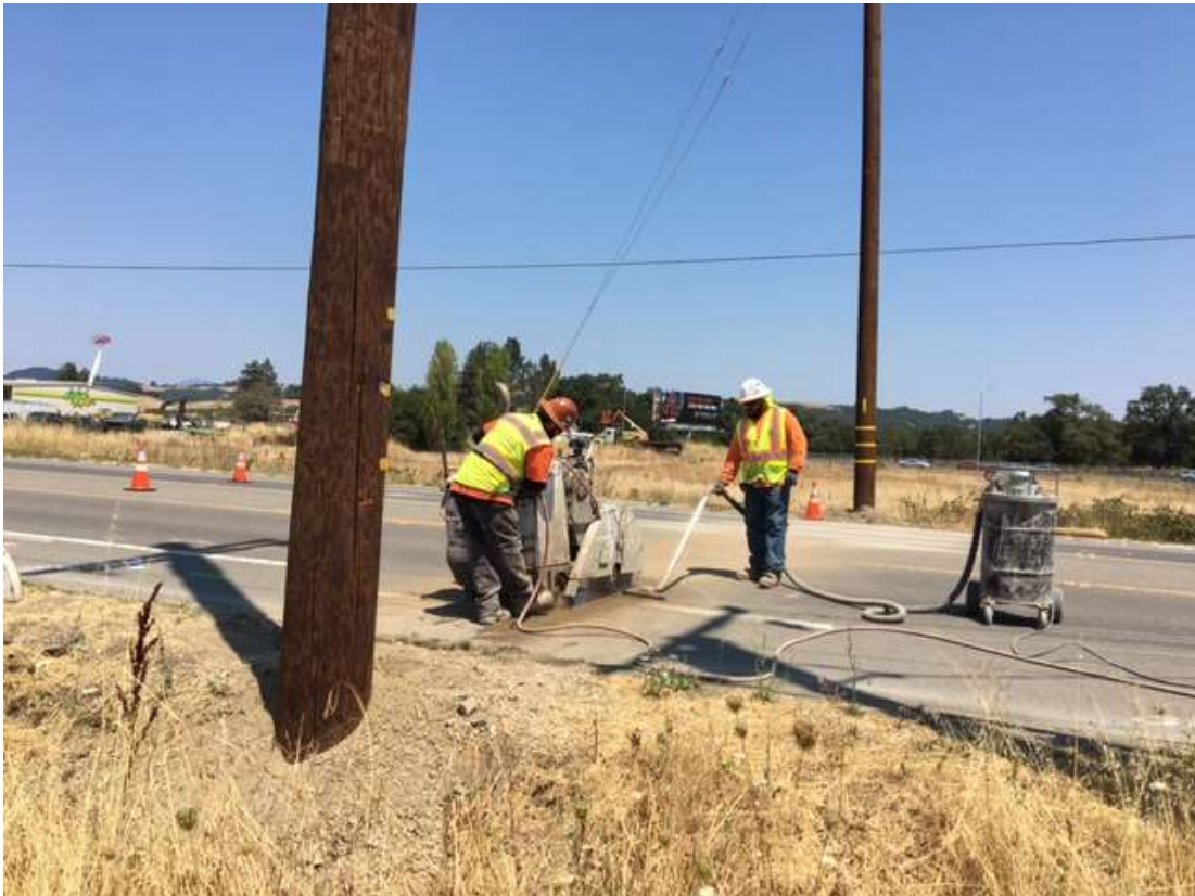
Figure 4 – Saw cutting across Old Redwood Highway – view east, August 1, 2017.
