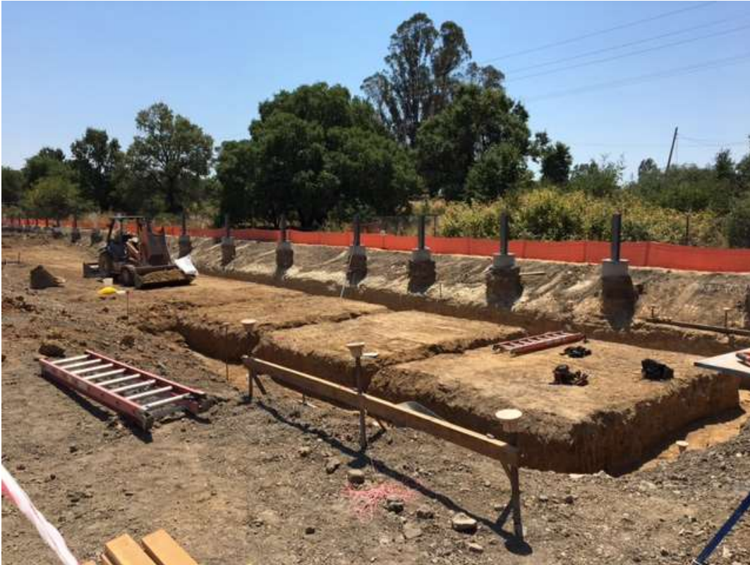
Figure 1 – SPCC pond excavation on west side of site – view southwest, August 1, 2017.
