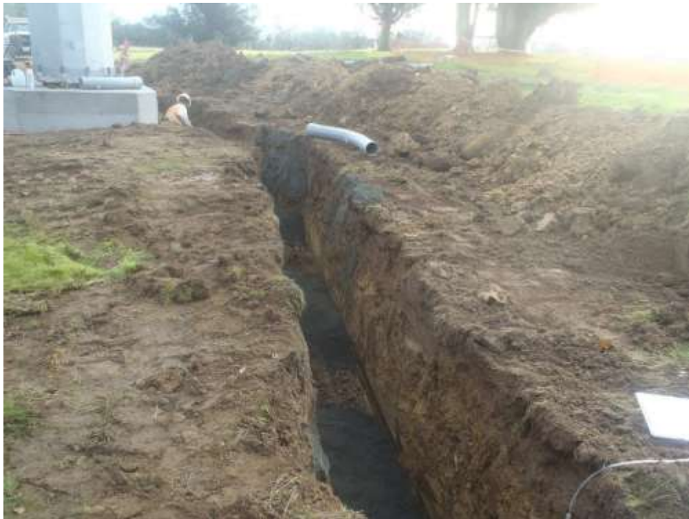
Figure 6 – Conduit trench to TSP – view south, December 27, 2017. Photo courtesy of PG&E.
