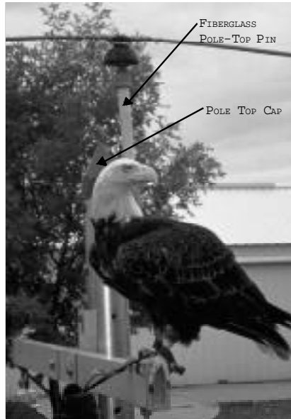
Photo 5. Distribution steel pole fitted with a pole-top cap to exclude perching.
