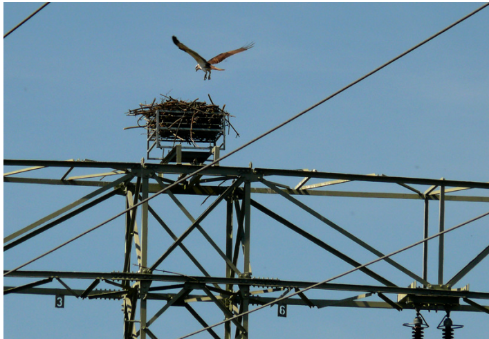
Figure 15. Nesting Osprey on artificial platform in medium voltage transmission line, Muritz National Park, Germany (Photo; Bureau Waardenburg).
