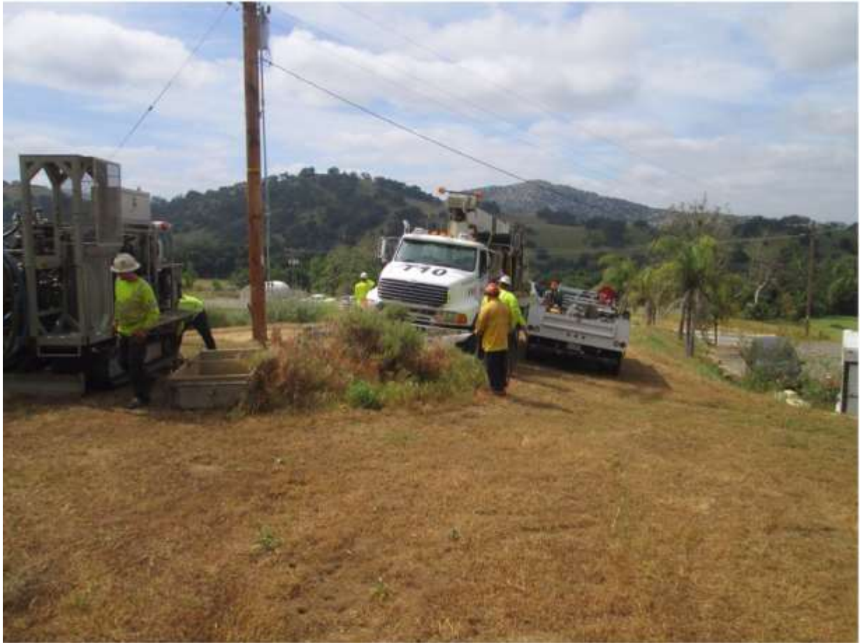
Photo 4: In accordance with CFPPP (MM FF-1), a fire patrol was observed pre-watering vegetation adjacent to a geotechnical drill at TL 682.
