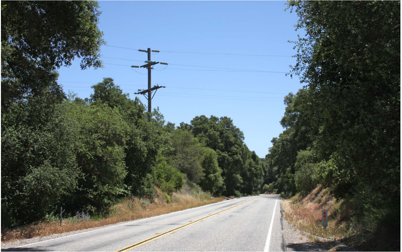
Existing view of Pole Z118144 from State Route 76 looking southeast.
