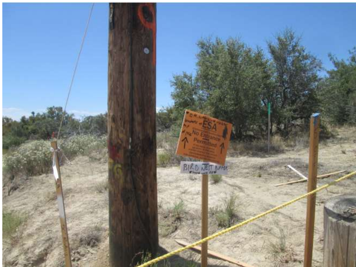
Photo 2: In accordance with MM BIO-28 and the NBMP, a nesting bird buffer was delineated at pole Z44242 (TL 6931). Approved avian monitors were observed surveying for nesting birds and checking buffers and status of nests throughout the right-of-ways.
