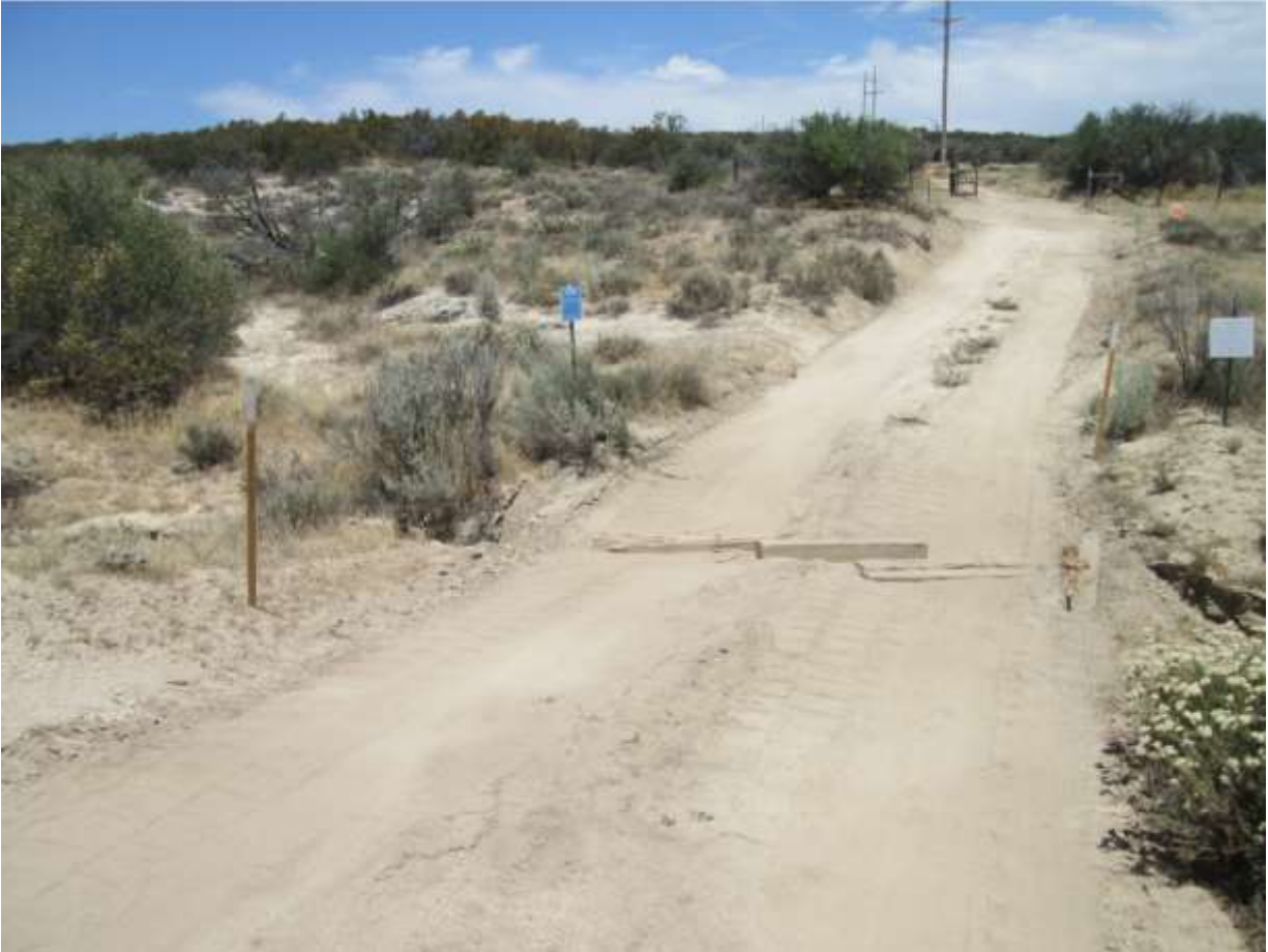
Photo 6: ESAs and markers indicating “No Grading, Water Crossing” were observed in place along TL 6931 (access road between Poles Z44245 to Z44246, above). “No grading” was also written on lath marking the water crossing.
