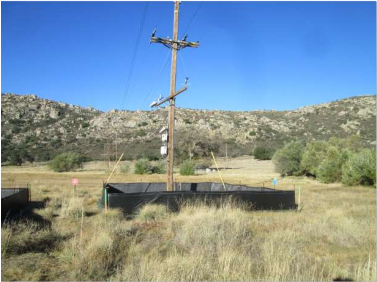
Photo 6: Protective fencing for arroyo toad in accordance with the Streambed Alteration Agreement measures for TL 629E was observed and areas were marked as ESAs for avoidance.
