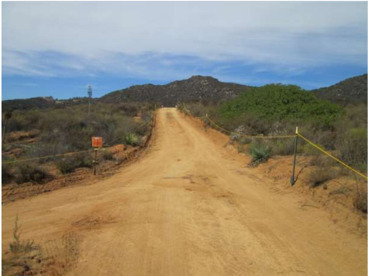
Photo 1: ESAs were observed marked for avoidance along TL 625B in accordance with APM CUL-03 and MM CUL-1/CUL-3.
