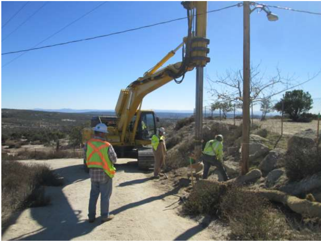
Photo 1: Crews were observed auguring a new pole location along TL 629E. Biological monitoring presence was observed in accordance with MM BIO-3.
