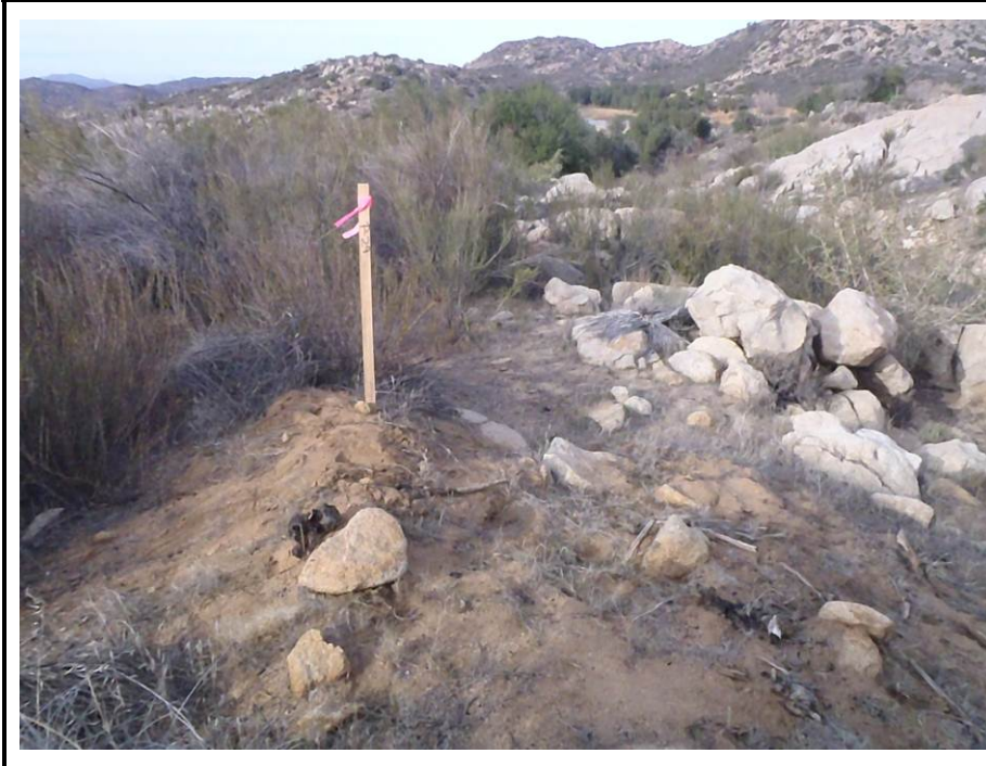
Photograph 5: View of pole P29 location west of Forest Route 17504 and south of an unnamed pond facing northeast.
