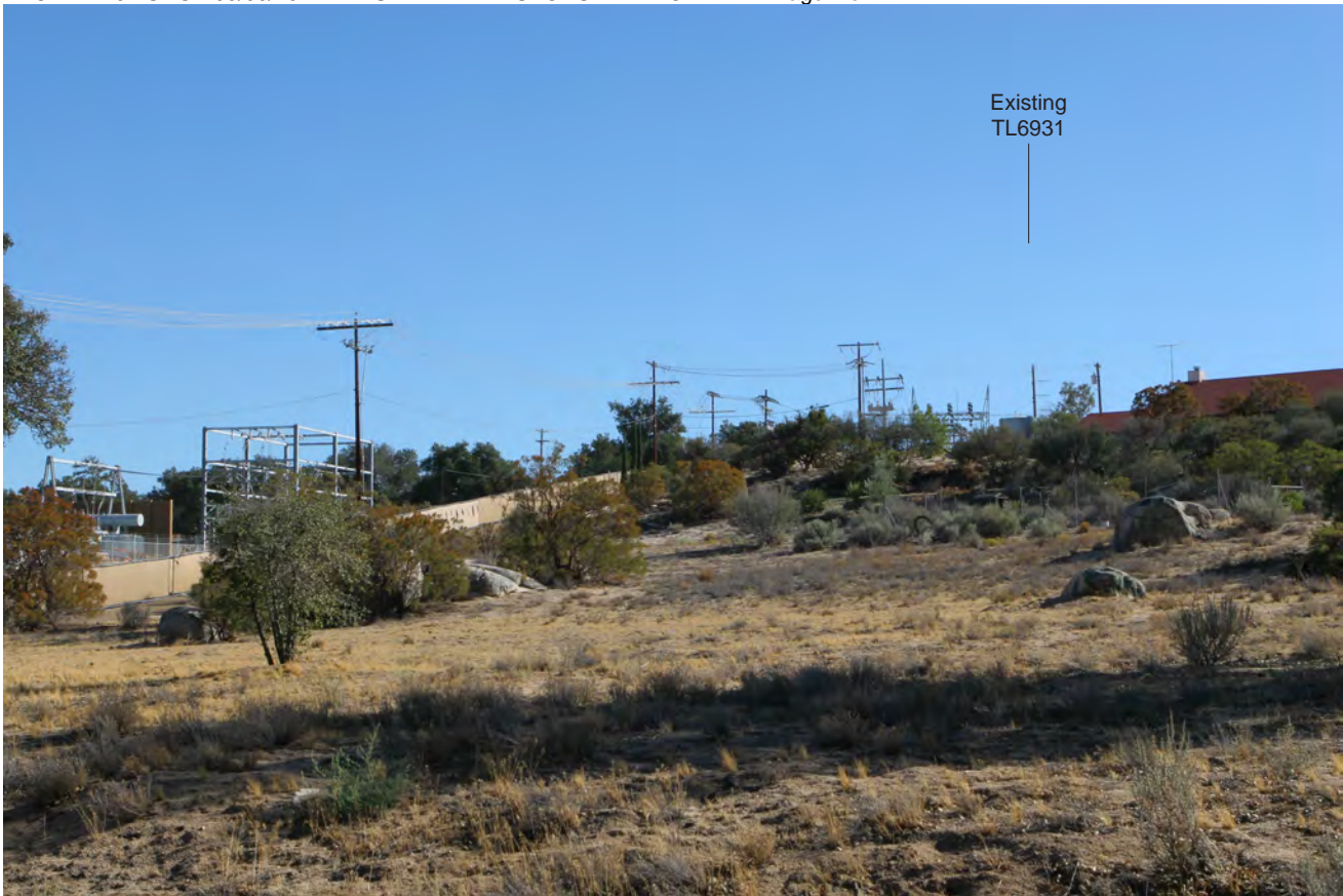
Existing view from Old Highway 80 at Boulevard Substation looking southeast (KOP 1)
