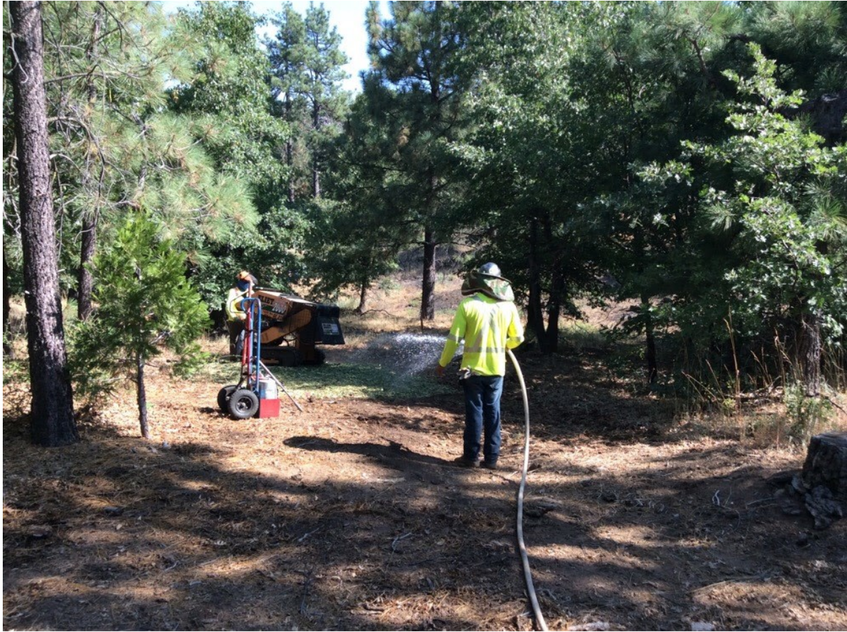
Photo 4: During vegetation chipping at Pole P260427 (C 440), a full set of fire tools was observed within 50 feet of the activity, at least 100 gallons of water with pump and hose were observed on site, and a crew member was observed wetting down the area in accordance with the CFPPP Fire Prevention Matrix for chipping on USFS land with a PAL C.
