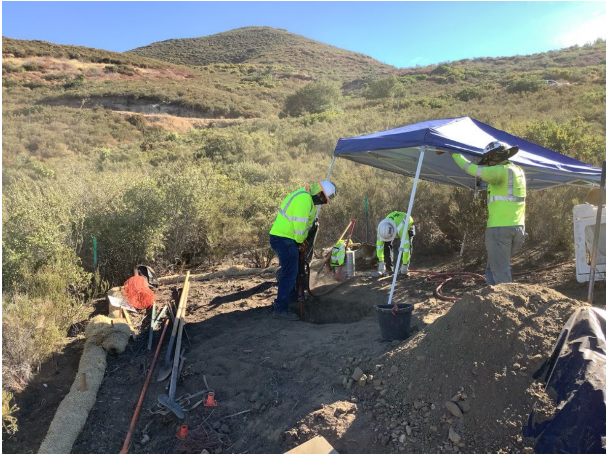
Photo 2: A crew was observed digging a direct bury pole hole at Pole P258496 (C 79B) within clearly delineated work limits in accordance with MM BIO-1.
