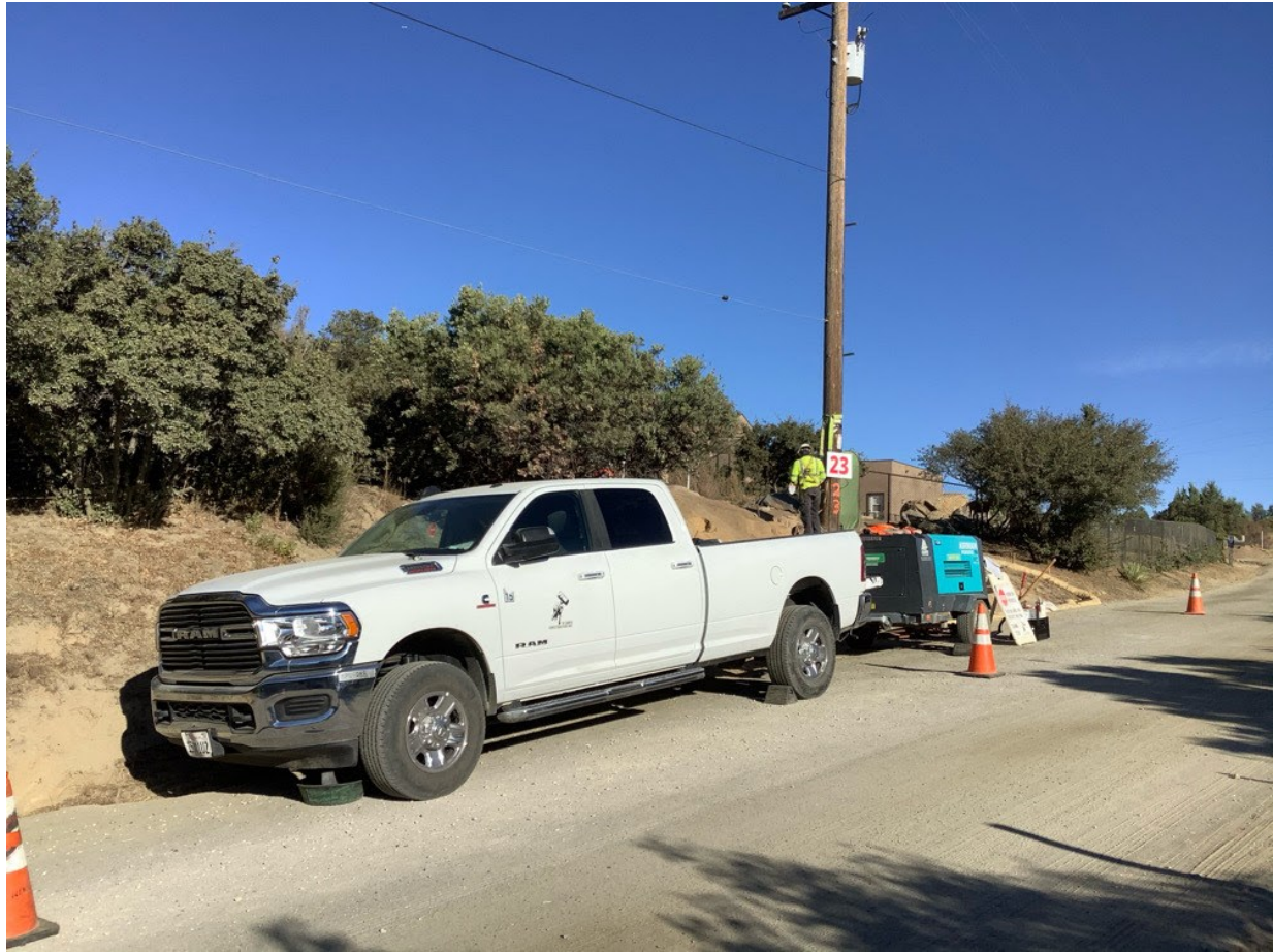
Photo 5: A drip pan was observed under a staged project vehicle at Pole P258472 (C 79B) to prevent leaks or spills from being discharged onto the ground in accordance with MM PHS-2.
