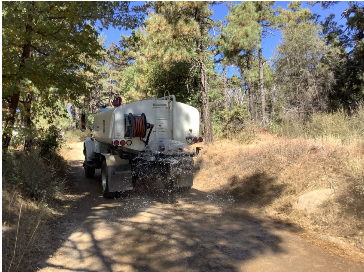
Photo 1: A water tender was observed applying water on Morris Ranch Road (C 440) to minimize dust emissions from Project vehicular traffic in accordance with APM AIR-02.
