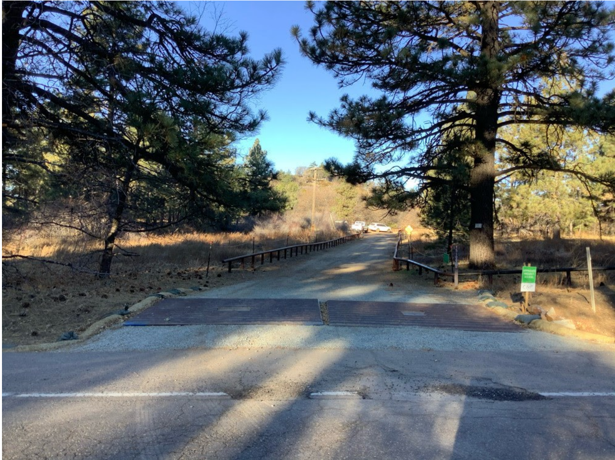
Photo 6: The entrance to Escondido Ravine Road (C 440) was observed to be stabilized with gravel and shaker plates to reduce trackout in accordance with the SWPPP (MM HYD-1 and MM BIO-7).
