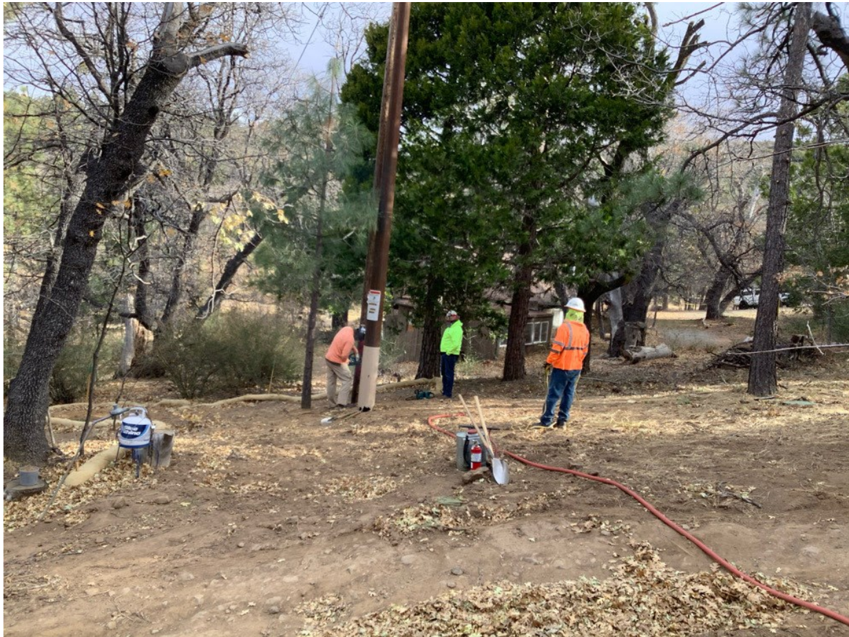
Photo 4: A crew was observed using a battery-powered chain saw to fell an old wooden pole at Pole P40443 (C 440). A full set of fire tools was observed within 50 feet of the activity in accordance with APM HAZ-04 and the CFPPP for hand tool use on NFS land with a PAL C.
