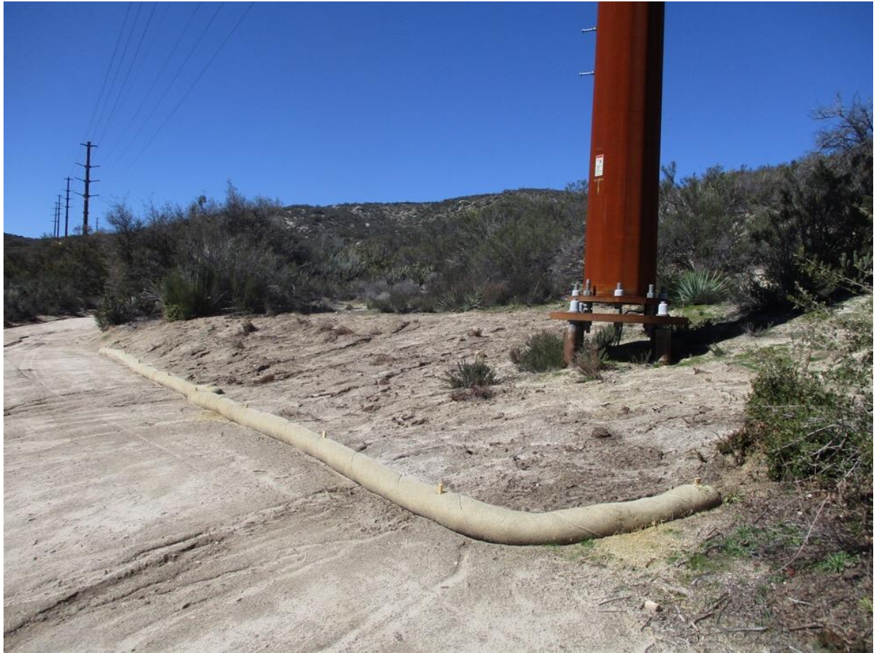
Photo 4: CPUC ECMs observed redistributed topsoil and a newly installed fiber roll for erosion and sediment control at the completed worksite at Z44201 (TL 629E).
