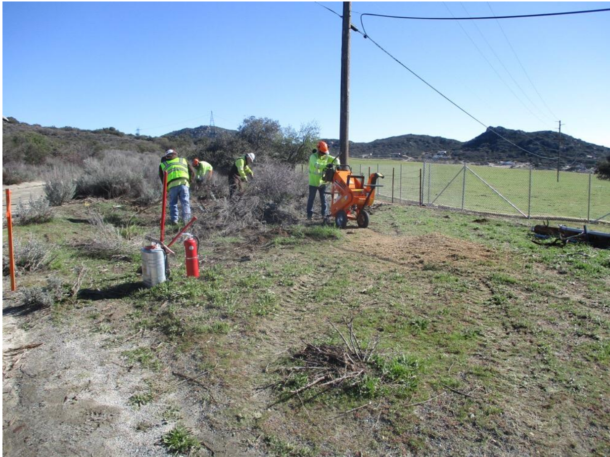
Photo 6: A complete set of fire tools was placed within 50 feet of the observed vegetation clearing and chipping activities at the southern entrance/exit to the Bartlett Staging Yard, in accordance with the CFPPP fire prevention matrix. A Biological Monitor was also observed monitoring the activities in accordance with MM BIO-3.
