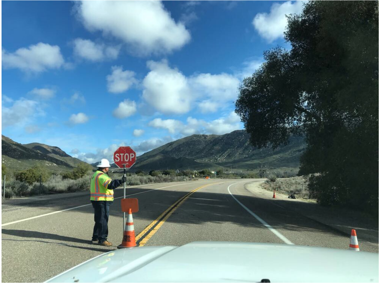
Photo 5: In accordance with APM TRANS-02, traffic was regulated on Buckman Springs Road (TL 629C) while helicopter external load operations were occurring across the road.
