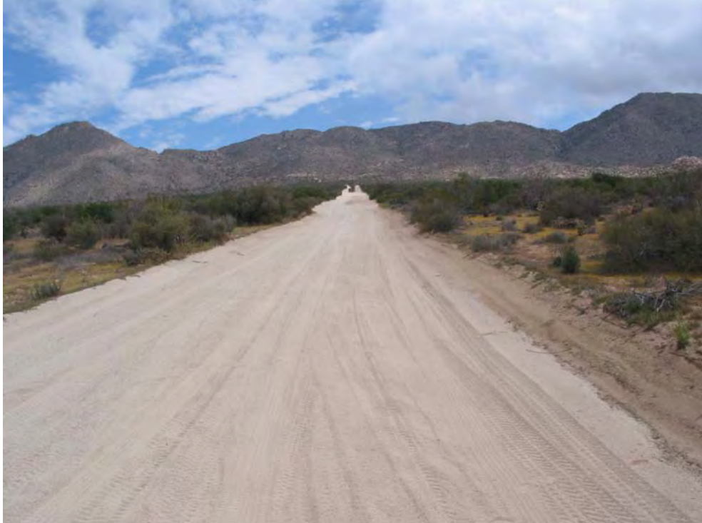
Photograph 9: View of existing east-west access road, looking east.
