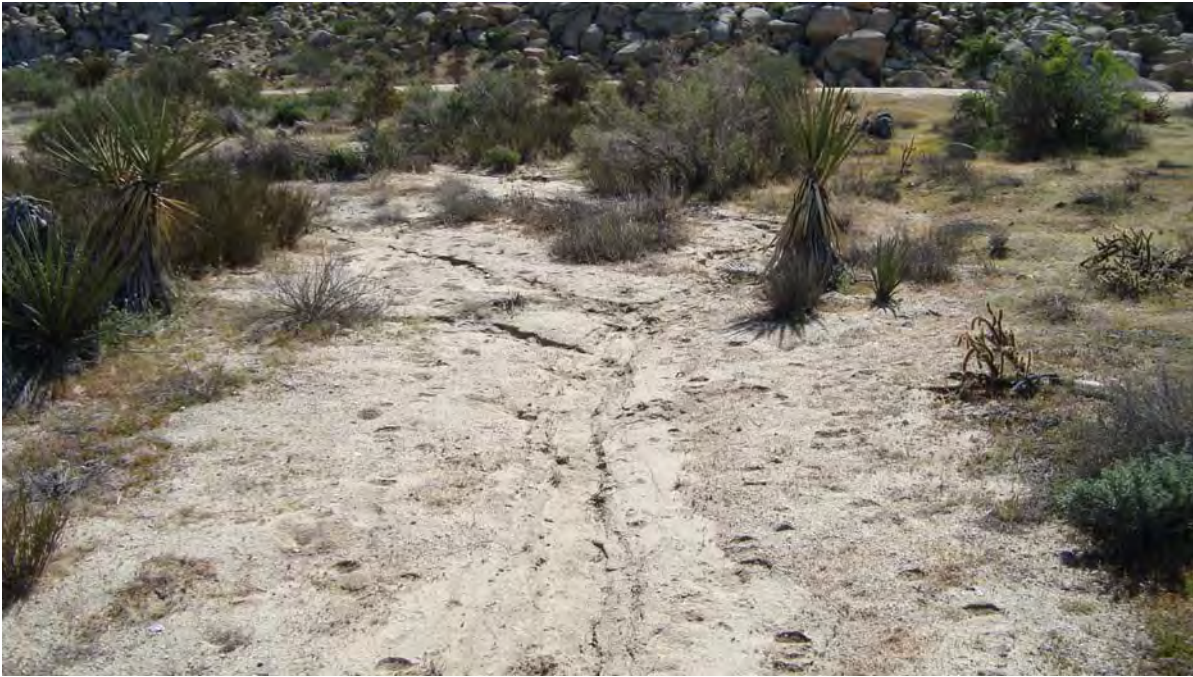
Photograph 1. View of southern erosive feature 1 looking east, with roadway in top background.
