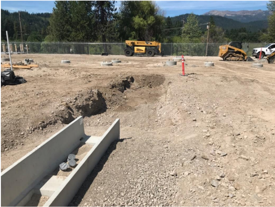
Photo 1: Excavated areas were ramped to prevent entrapment (APM BIO-6).
