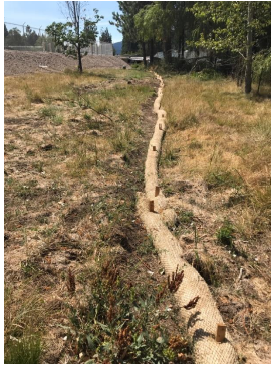
Photo 3: SWPPP erosion control BMPs (fiber rolls) were observed in good condition along the project boundary in accordance with APM WQ-1.
