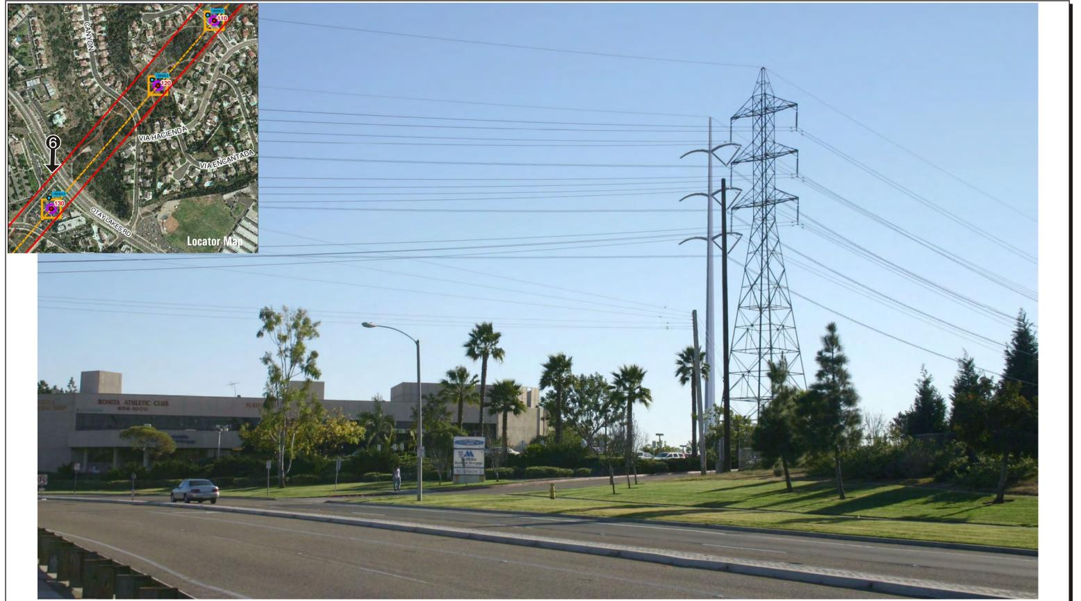
The proposed 230kV monopole structure (No. 130) and conductors are shown in this **visual simulation**. Located slightly farther from the viewer, the proposed 140' tall monopole structure appears similar, or slightly smaller in scale than the 125' tall lattice tower. The proposed monopole would be visually dominant with the existing lattice structure. Visual contrasts would be strong, although viewing duration would be short-term and transient in nature.
