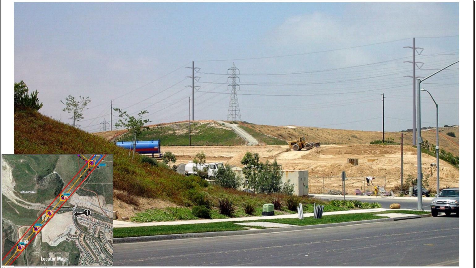
The proposed 230kV monopole structures (No. 30 and 40) and conductors are shown in this **visual simulation**. The closest proposed structure, No. 30, would be 145' in height, compared to the 107' tall existing lattice tower. Located adjacent to viewers on the elevated hill, the proposed monopoles and conductors would be visually dominant with the existing lattice structures and lines, and would create strong visual contrasts.
