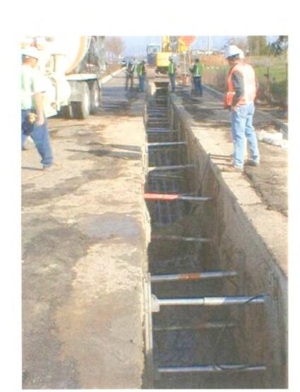
Trench in street. Conduit for individual transmission cables visible in center of photo.
