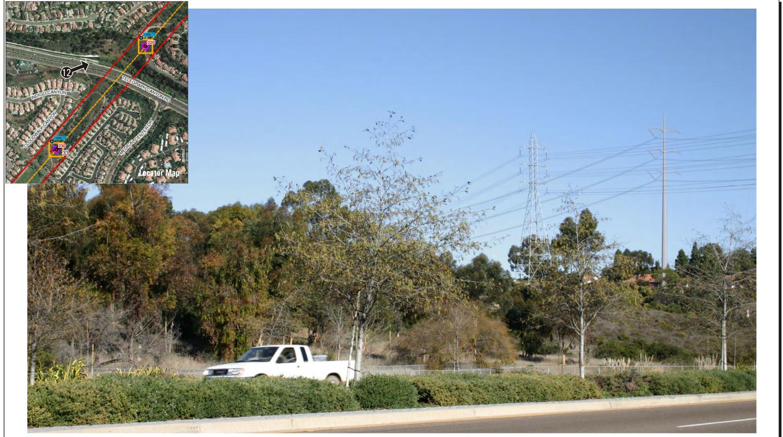
The proposed 230kV monopole structure (No. 220) and conductors are shown in this visual simulation. The monopole would be located slightly farther from the viewer, although the proposed 155' tall monopole structure would appear larger in scale than the 125' tall lattice tower, due to both increased structure height and base elevation. The proposed monopole would be visually dominant with the existing lattice structure.
