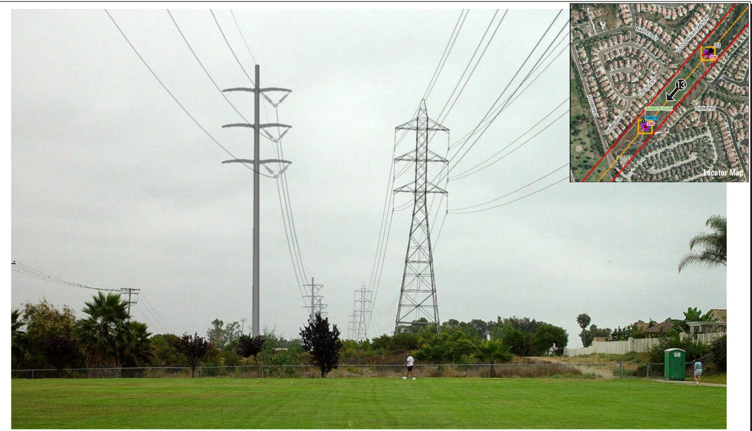
The proposed 230kV monopole structures (No. 240, 250 and 260) and conductors are shown in this visual simulation. The proposed structures would range in height from 125' to 145', compared to the existing lattice towers that are between 107' to 120' tall. Located over the park, the proposed monopoles and 230kV conductor would be visually dominant, and in conjunction with the existing 138kV lattice facilities, create very strong visual contrasts.
