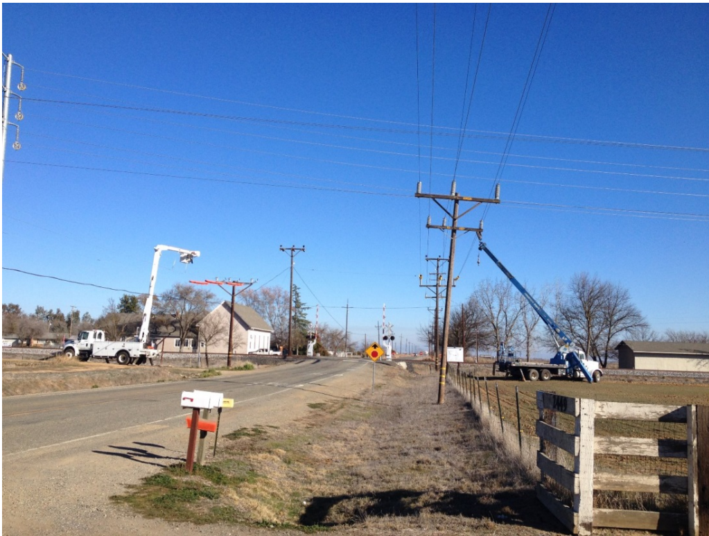
Figure 2: Bucket truck as guard structure.
