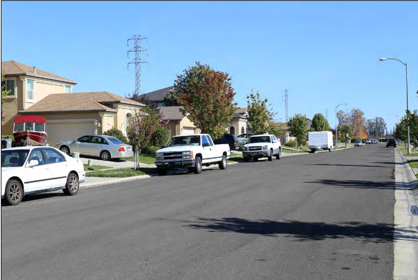
Existing view of the Bogue Single-Circuit Sub-Line Segment from Chateau Drive
