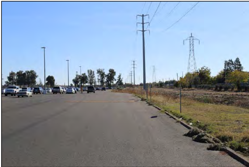
Photograph 13 - View of South of Palermo Single-Circuit Line and adjacent power line from Yuba College campus (Marysville)
