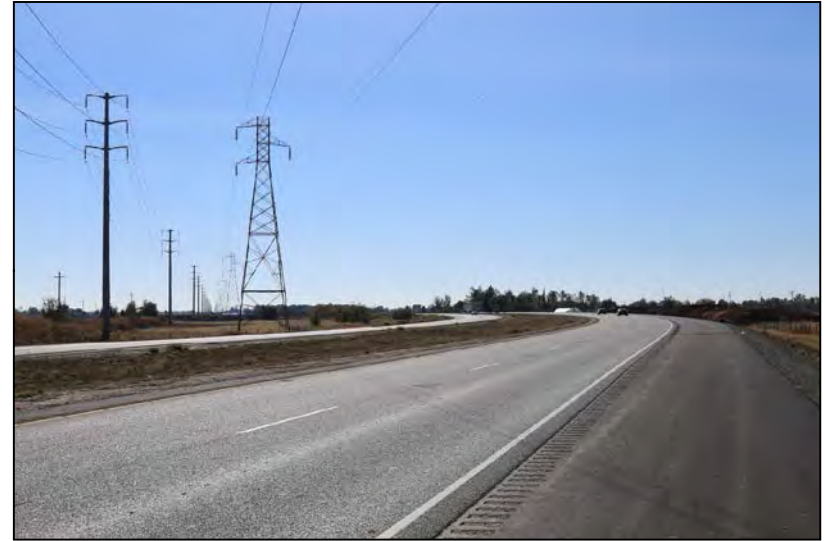
Photograph 22 - View of South of Palermo Single-Circuit Line and adjacent power line from SR-70 (Olivehurst)
