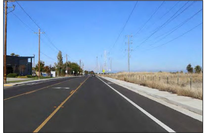
Photograph 18 - View of South of Palermo Single-Circuit Line and adjacent power line from Powerline Road (Olivehurst)
