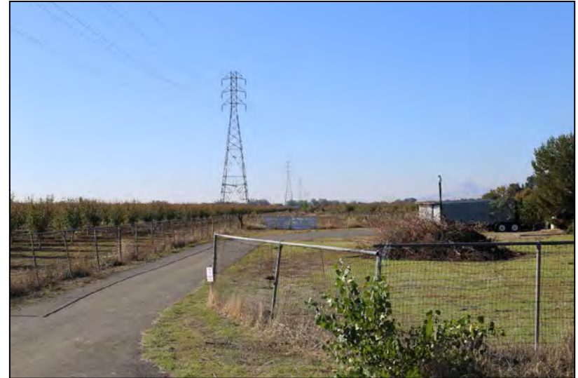
Photograph 10 - View of Pease Single-Circuit Sub-Line Segment from SR-70 (Marysville)
