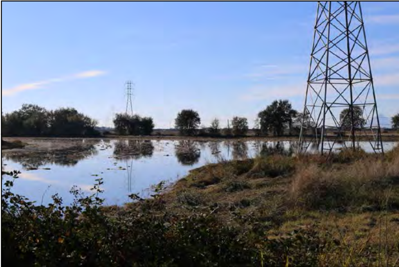
Photograph 9 - View of Pease Single-Circuit Sub-Line Segment from Jack Slough Road (Marysville)
