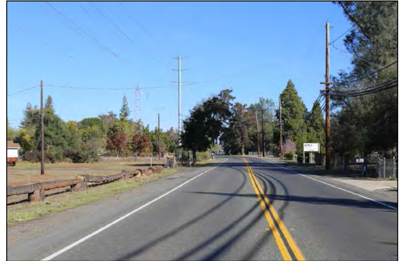
Photograph 2 - View of South of Palermo Single-Circuit Line and existing utilities from Lincoln Boulevard (Palermo)
