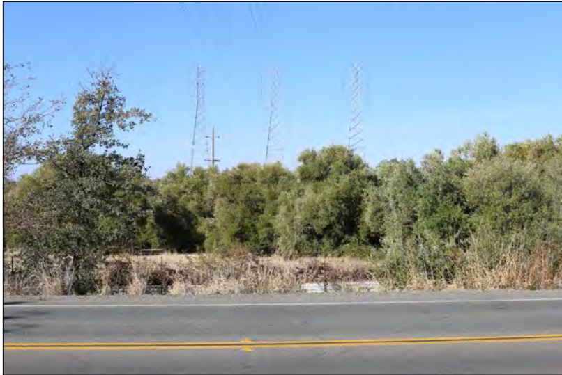
Photograph 1 - View of Palermo Double-Circuit Sub-Line and adjacent power lines from Upper Palermo Road
