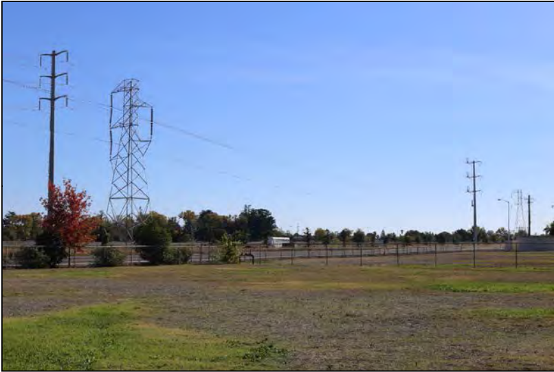
Photograph 17 - View of South of Palermo Single-Circuit Line and adjacent power line from 9th Avenue (Olivehurst)
