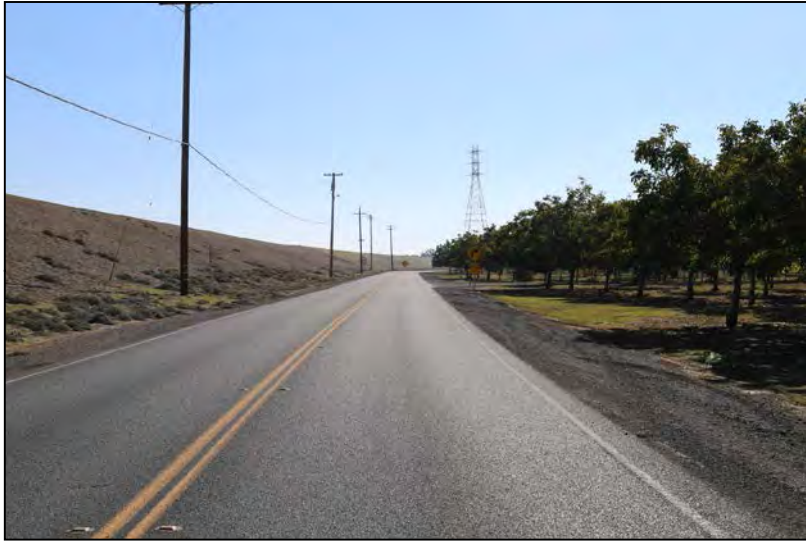
Photograph 21 - View of Bogue Single-Circuit Sub-Line Segment and distribution line from Garden Highway (South Yuba City area)
