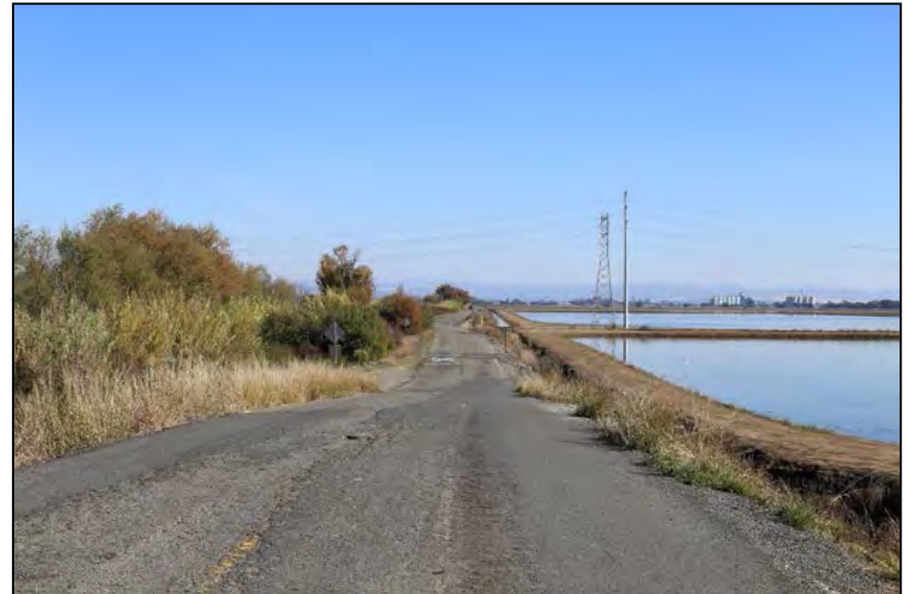
Photograph 8 - View of South of Palermo Single-Circuit Line and adjacent power line from Woodruff Lane (North Yuba County)
