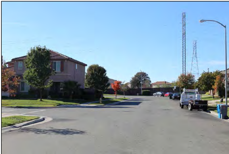
Photograph 15 - View of South of Palermo Single-Circuit Line and adjacent power line from Waterville Drive (Marysville)
