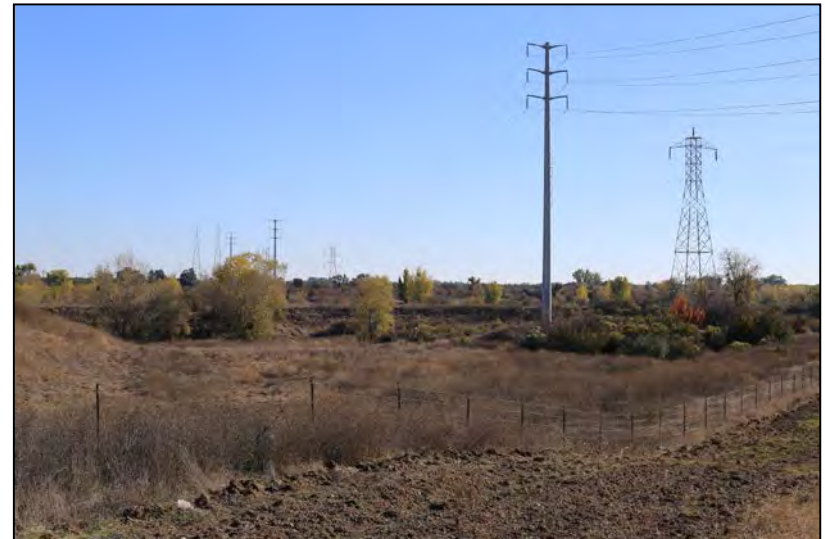
Photograph 12 - View of South of Palermo Single-Circuit Line and adjacent power line from SR-20 (Marysville)
