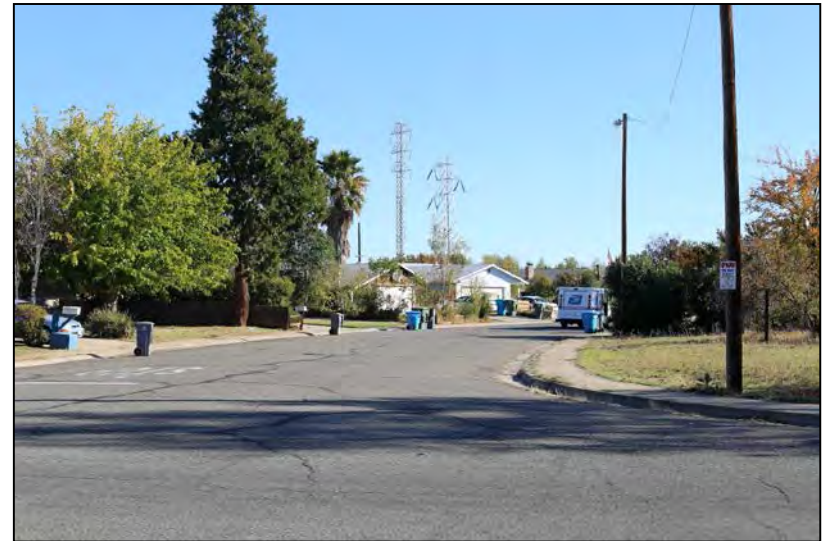
Photograph 14 - View of South of Palermo Single-Circuit Line and adjacent power line from Wildwood Drive (Marysville)
