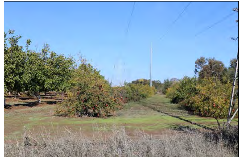
Photograph 24 - View of South of Palermo Single-Circuit Line and adjacent power line from Rio Oso Road (Rio Oso)
