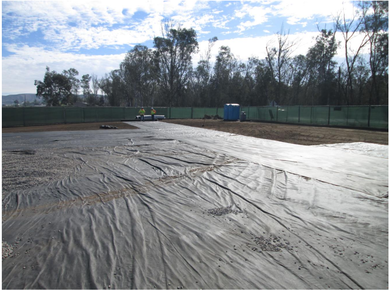
Photo 3: Mirafi material was observed placed on the surface of the Warnock Staging Yard prior to gravel installation in accordance with BMPs for erosion and sediment control.
