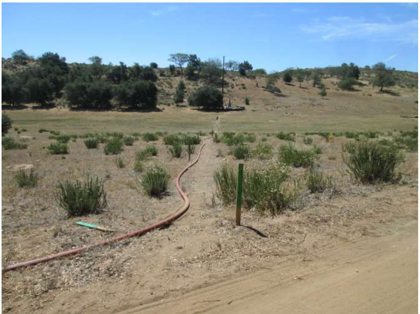
Photo 6: In accordance with MM-HYD-2 and the 401 Permit Certification, construction personnel were observed using a footpath to access Structure No. P106 to minimize impacts to the wet meadow between the location and the main access road. High pressure hoses connecting the compressor to the drill rig was laid down along the footpath.
