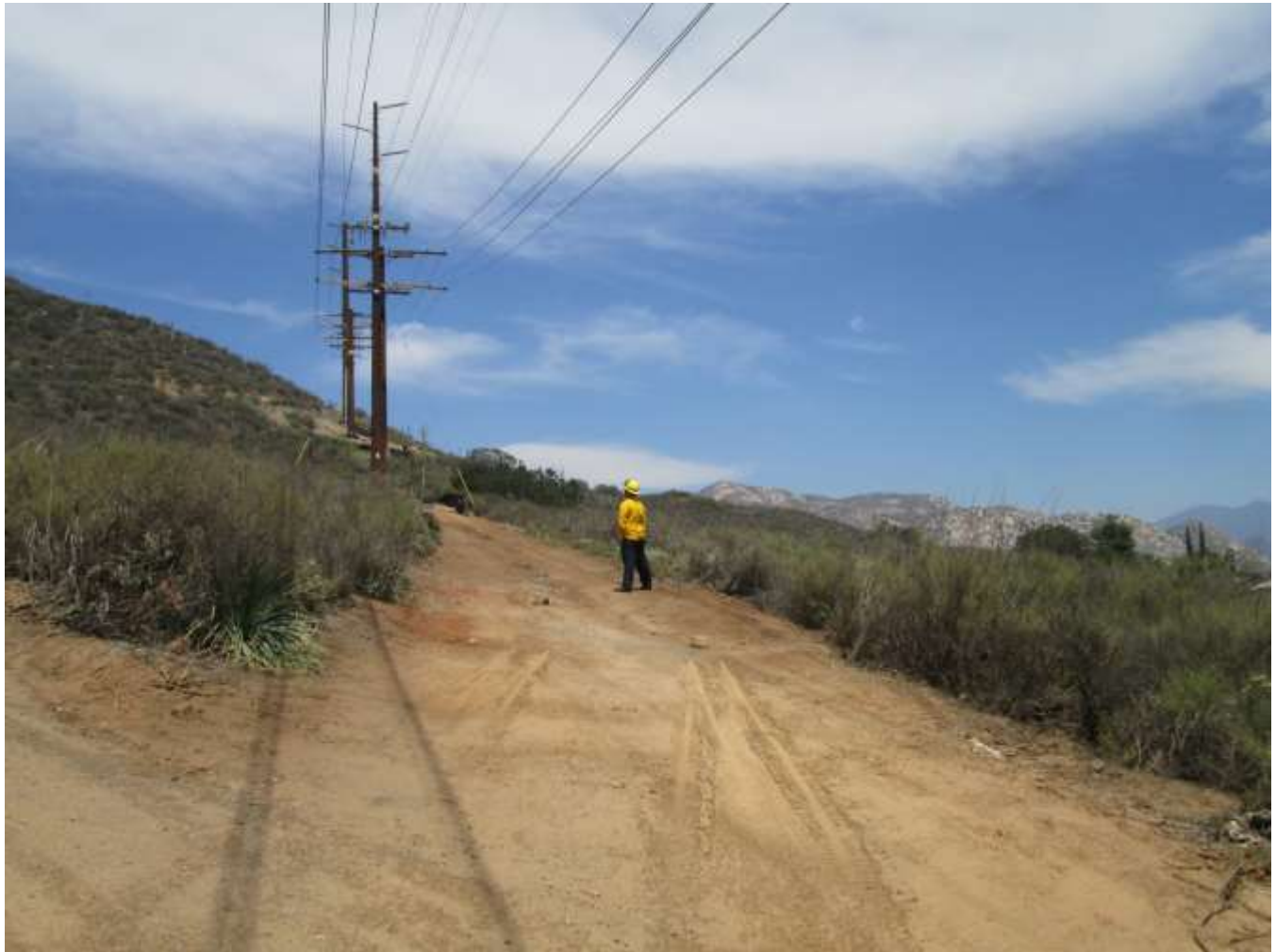
Photo 7: In accordance with the Project Fire Plan and APM HAZ-2, fire patrols were observed monitoring construction activities and inspecting work locations for fire safety compliance.
