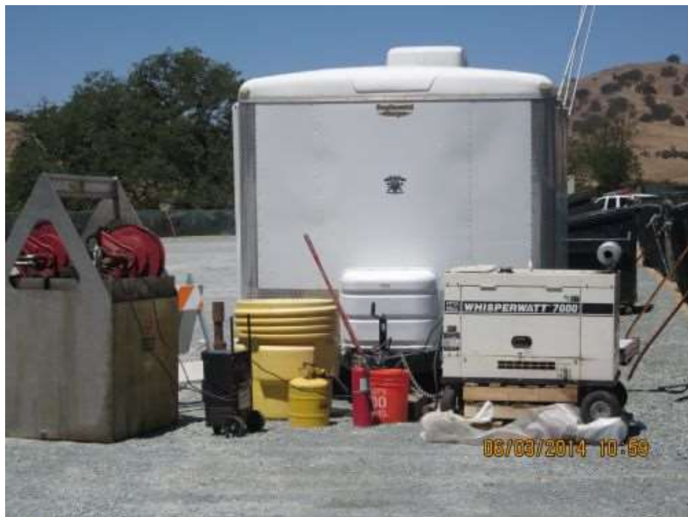
Photo 4: Fire tools and spill kits were staged at the Santa Ysabel Staging Yard and visqueen was staged under equipment to prevent potential soil contamination in accordance with APM HAZ-2.
