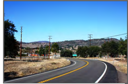
Existing wood TL 637 and TL 626 double-circuit structure south of Santa Ysabel Substation (two structures in foreground supporting a double-circuit configuration)
