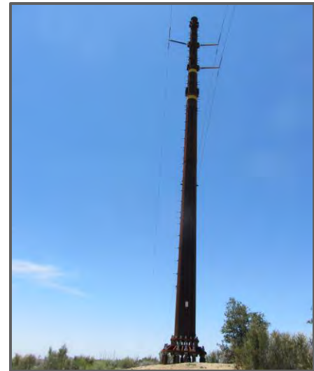
TL 637 steel pole on Cleveland National Forest jurisdictional lands (P116 – micropile foundation)
