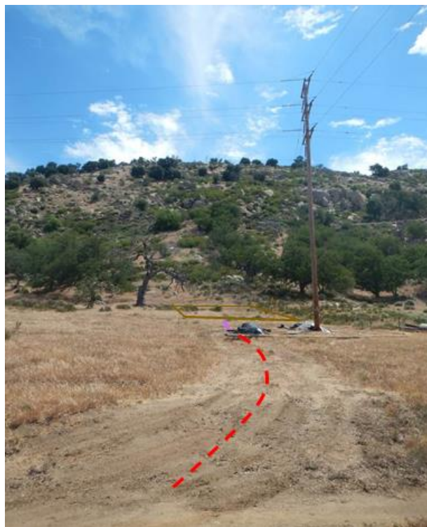
Photograph 5: Proposed overland travel route (purple) past P151 to SS-21 (outlined in brown), with existing road access to P151 shown in red, facing northeast.
