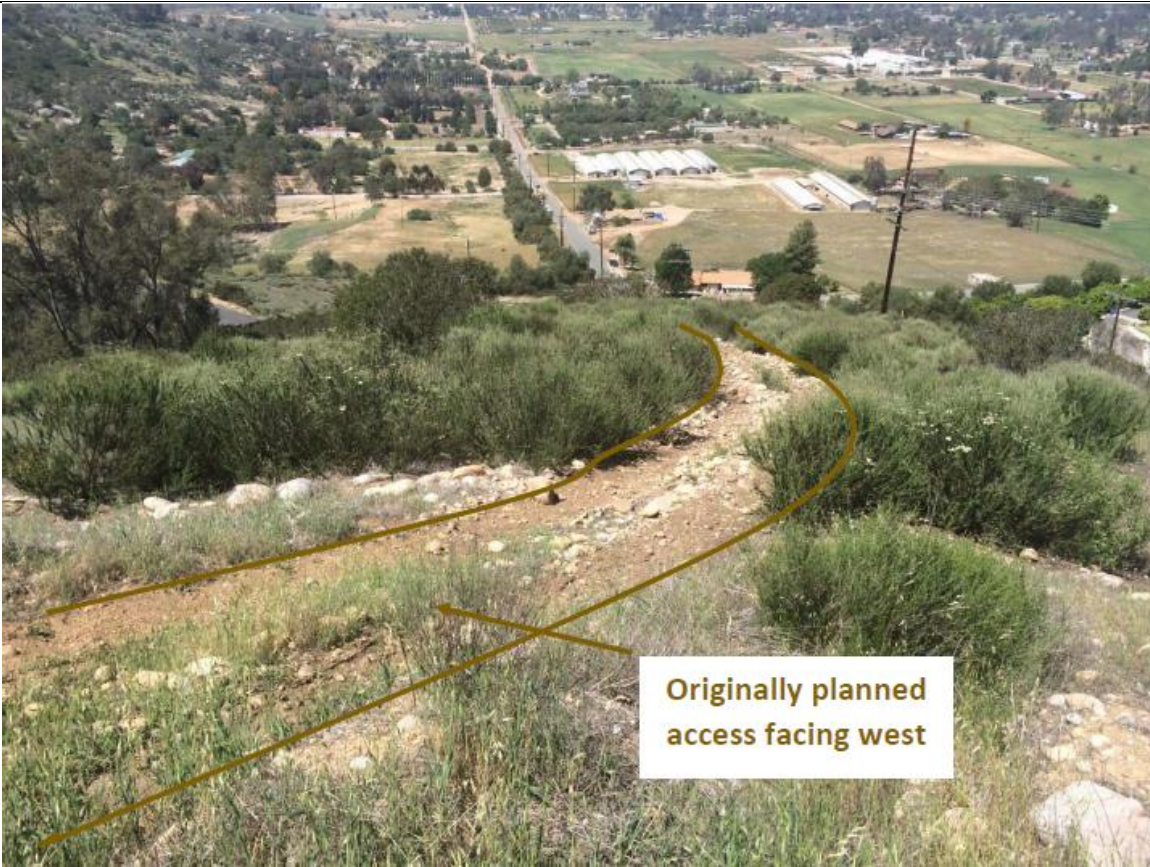
Photograph 1: View of Original Access Road facing West
