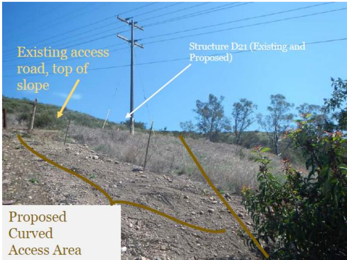
Photograph 4: View of area for curved access area where overland travel route intersects existing access road, facing southeast.
