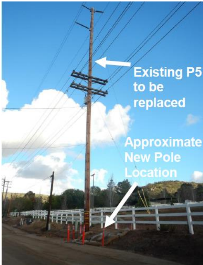
Photograph 1: Existing location Structure No. P5 facing southeast
