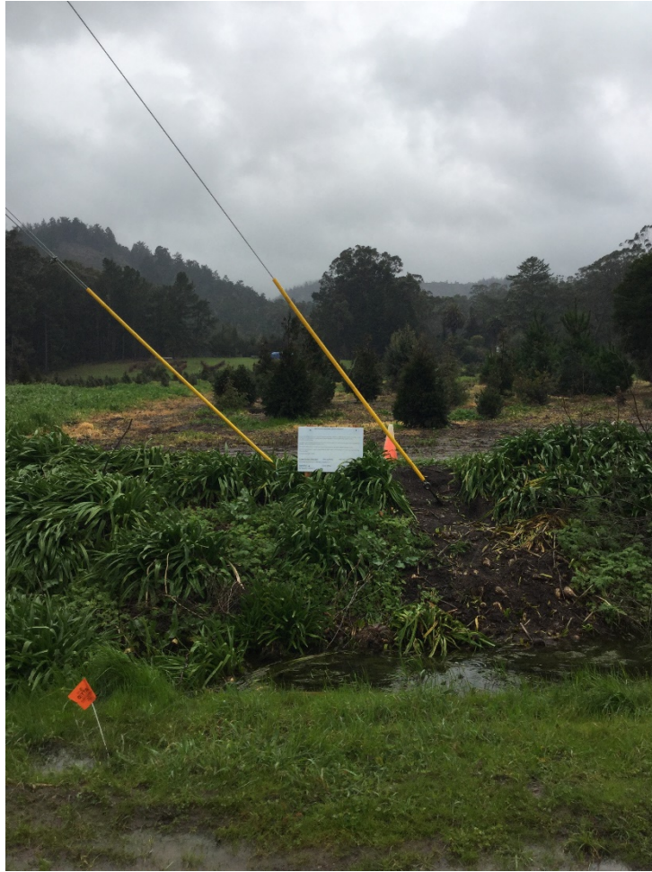
Photo 2: Pole anchors and project notification sign.
