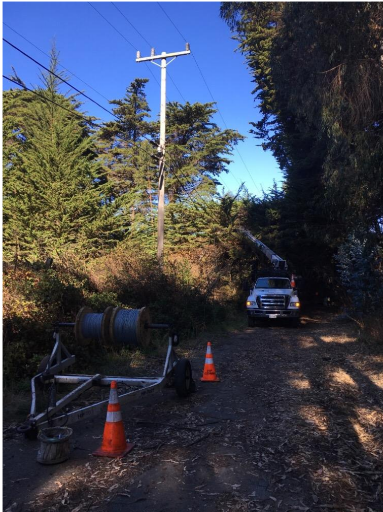
Photo 5: Aerial crew bucket rig and active installation operations.
