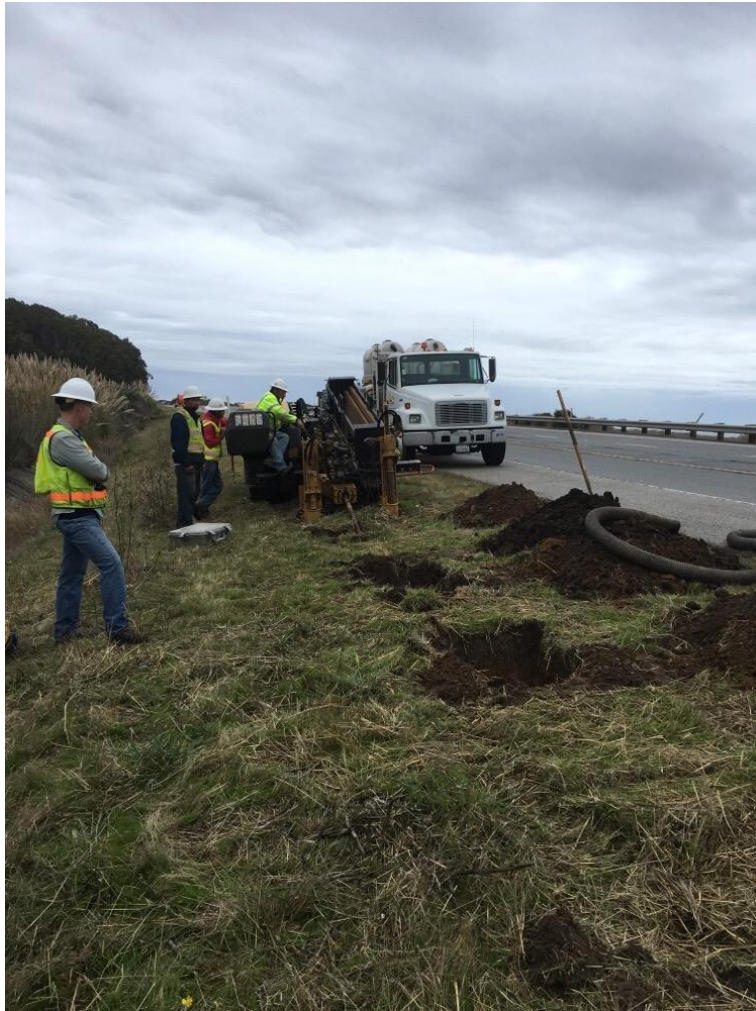
Photo 7: Active HDD installation along Highway 1, northbound at mile marker 5.2.
