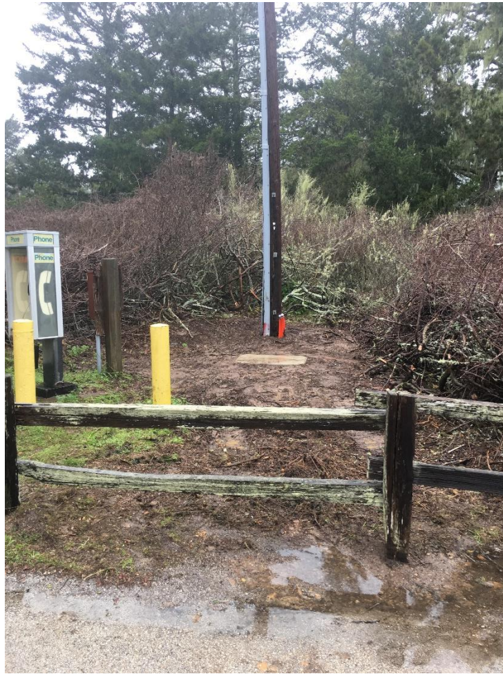
Photo 7: Newly installed utility box near Año Nuevo State Park.
