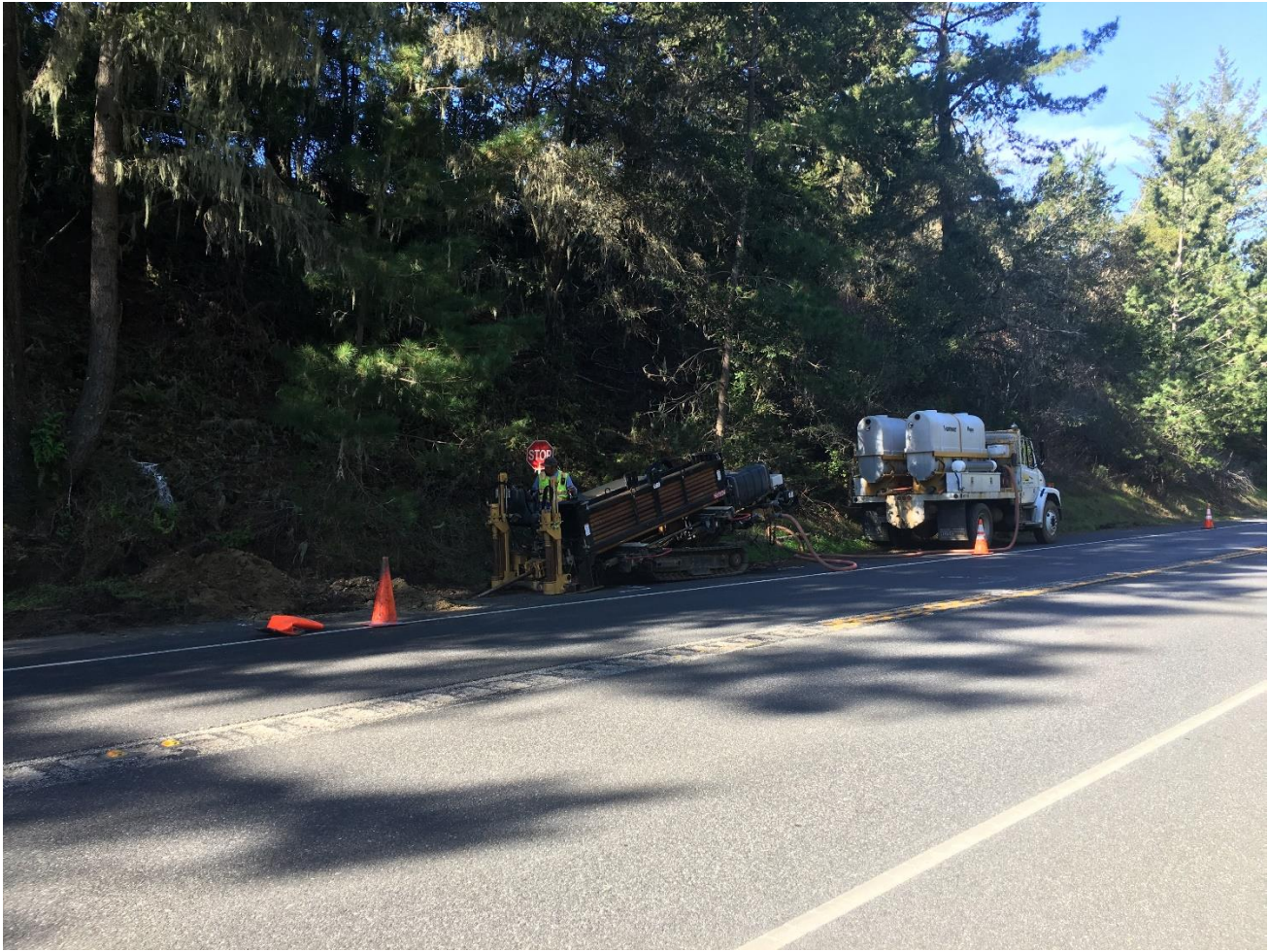
Photo 3: Horizontal Directional Drill (HDD) operations along Highway 1 southbound shoulder.
