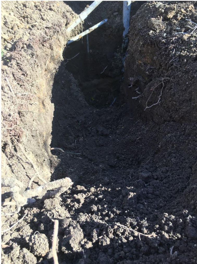
Photo 5: Excavation to prepare underground/aerial union near Año Nuevo State Park.
