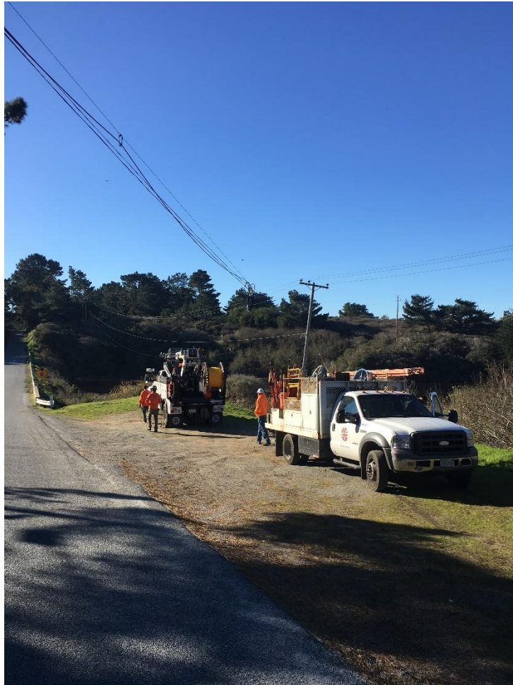
Photo 1: Aerial fiber-optic line installation along Bean Hollow Road.
