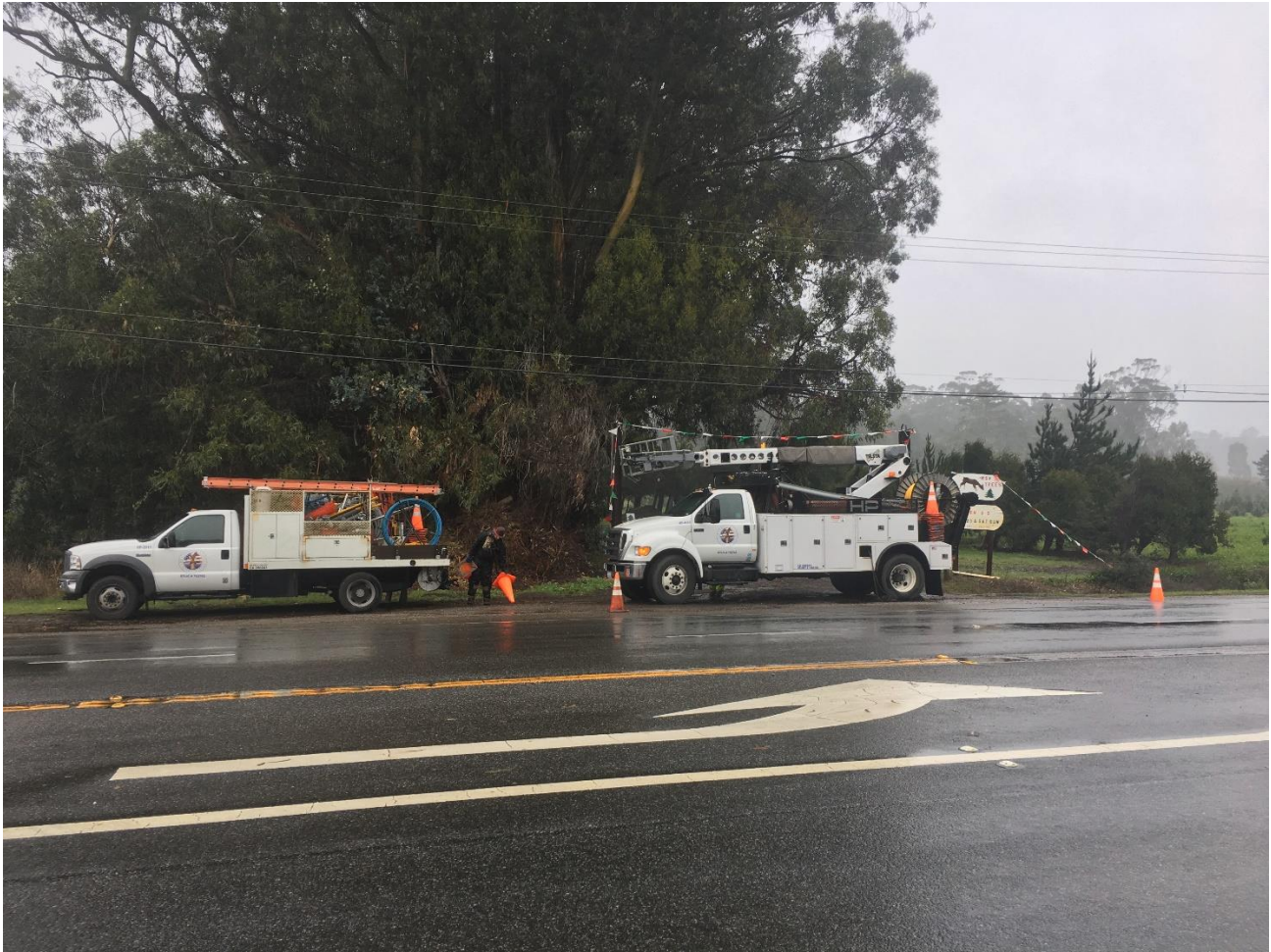
Photo 6: Aerial fiber-optic line installation.
