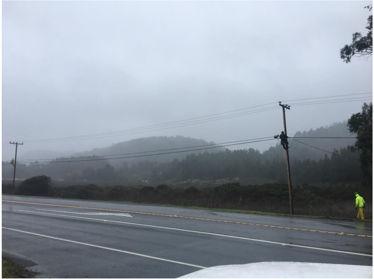
Photo 8: Aerial fiber-optic line installation.
