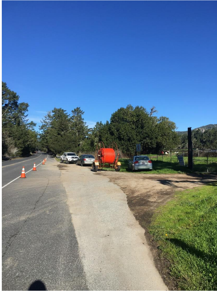
Photo 2: Parking and conduit materials staging along Highway 1 northbound.
