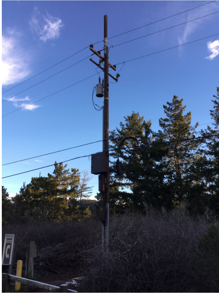
Photo 2: Fiber optic line installation complete at this pole location.
