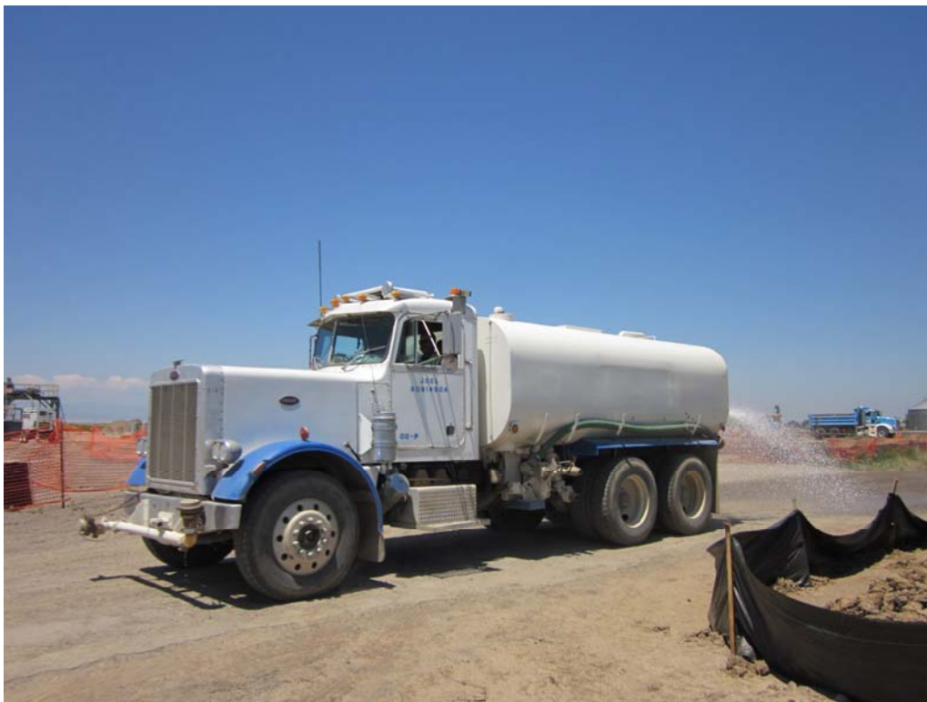
Photo 5: Dust control measures being implemented at the remote well pad site.
