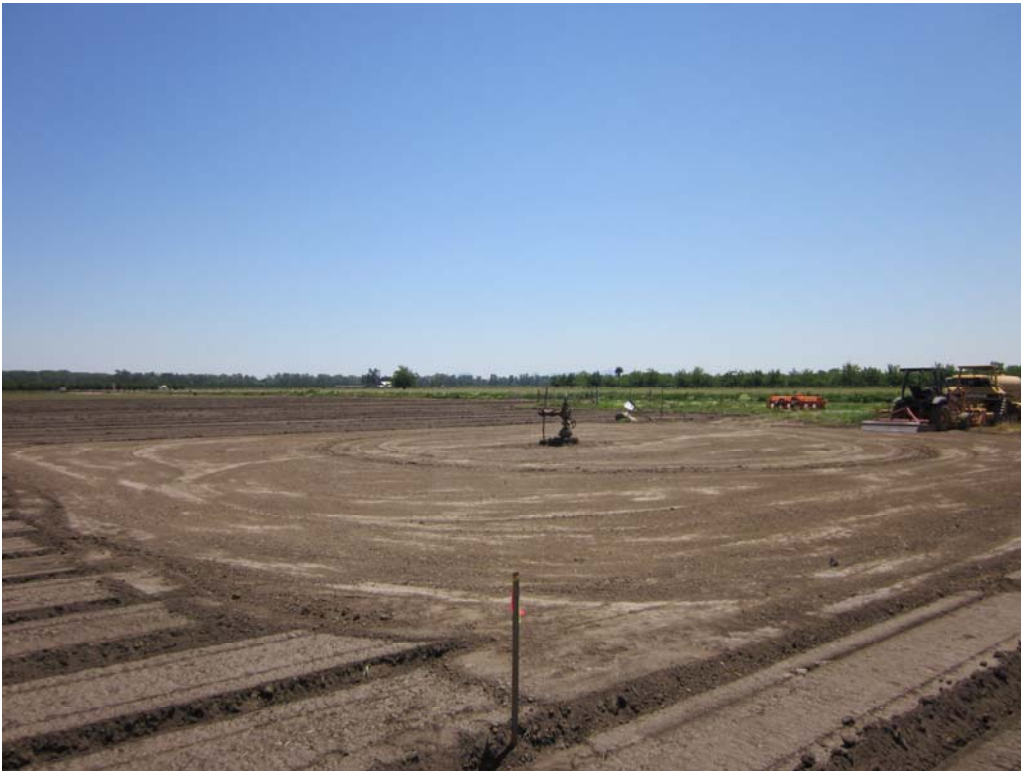
Photo 4: Graded area at the Southam #3 observation well.
