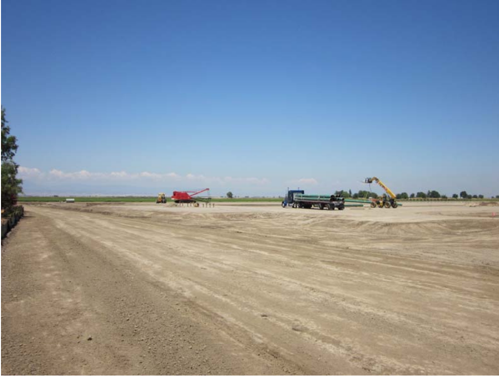
Photo 3: Completed grading at the compressor station site. Note silt fence intact at edge of construction area (at left edge of photo).
