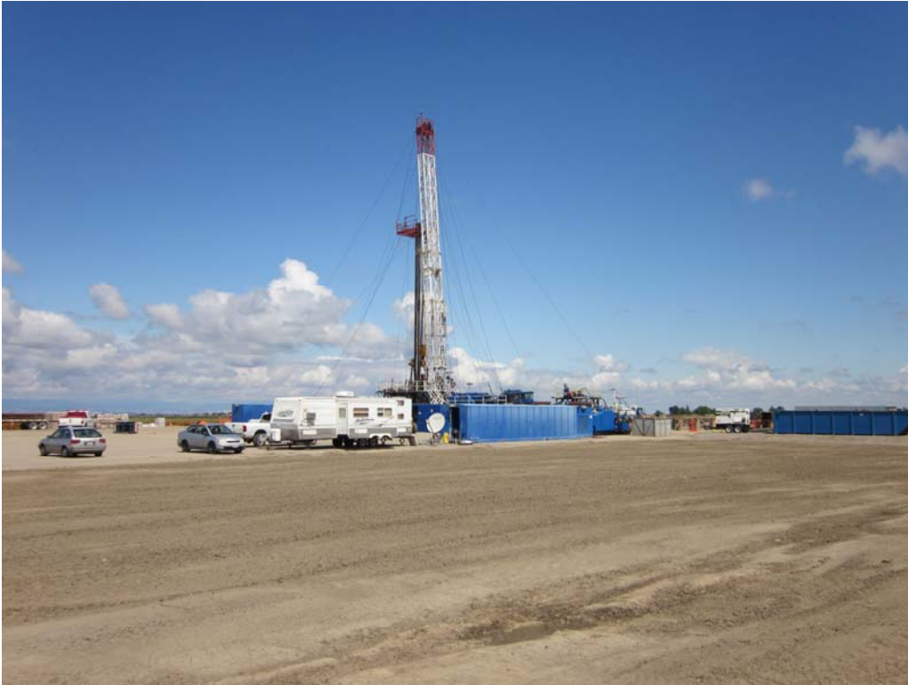
Photo 1: Drilling rig set up at the remote well pad site.
