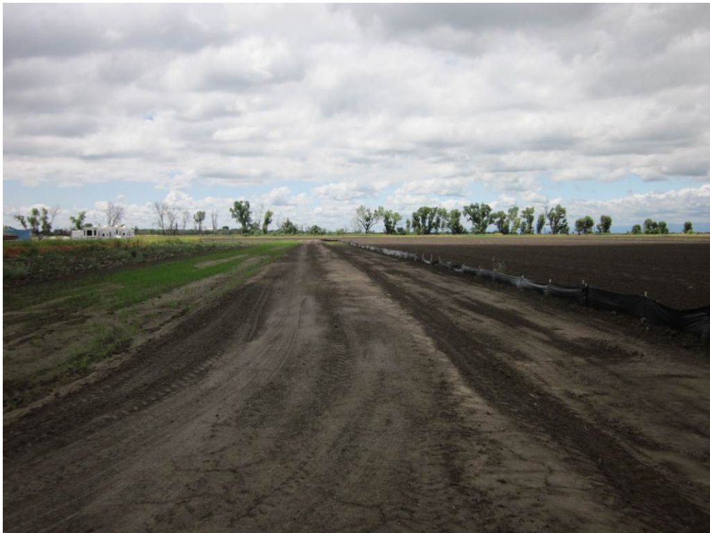
Photo 6: Exclusion fencing and silt fencing at the western edge of the remote well pad site to ensure protection of sensitive habitats.
