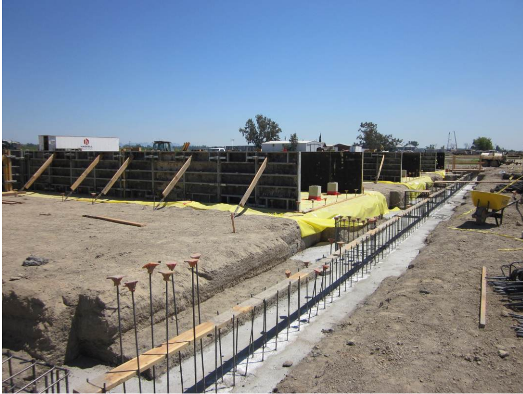
Photo 5: Building foundation work at the compressor station site.
