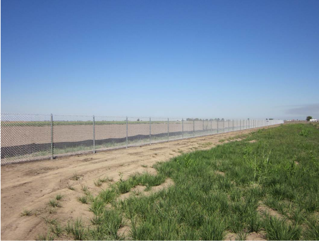
Photo 3: Permanent fence installation at the remote well pad site.
