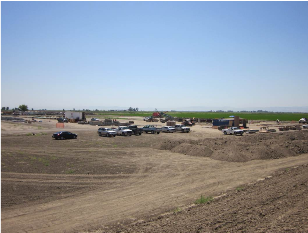
Photo 4: Building foundation work at the compressor station site.
