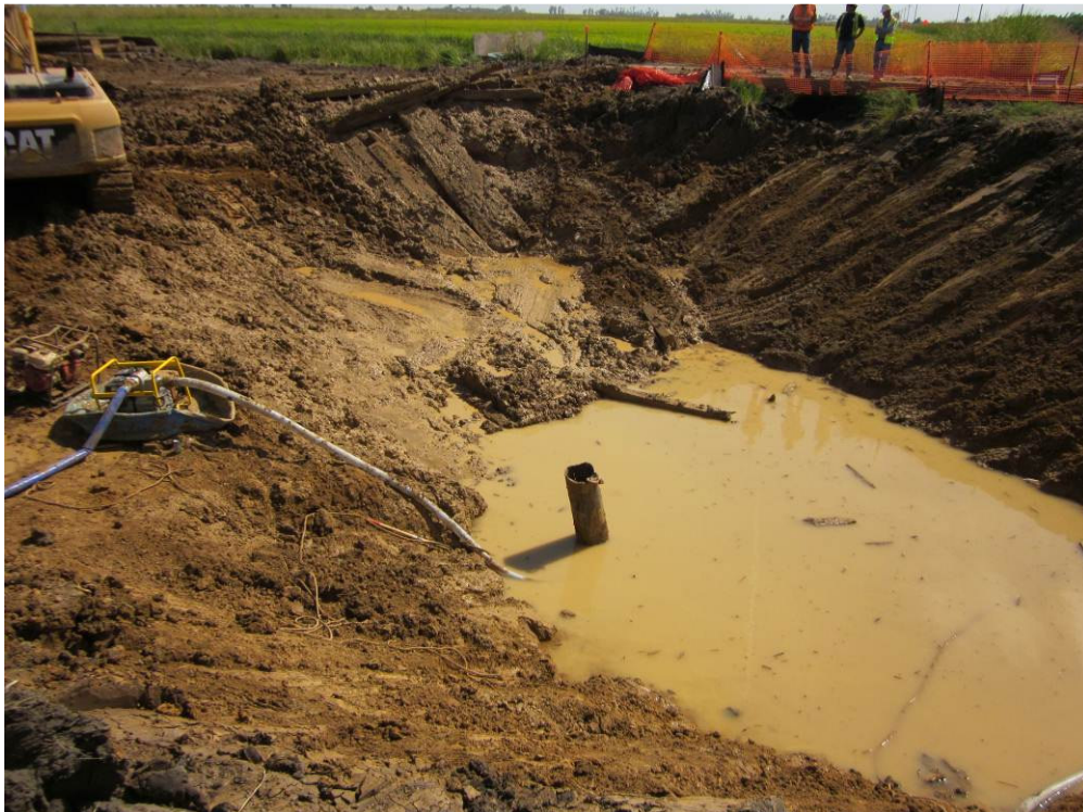
Photo 2: Auger bore hole excavation and dewatering at the Dirks Road crossing.
