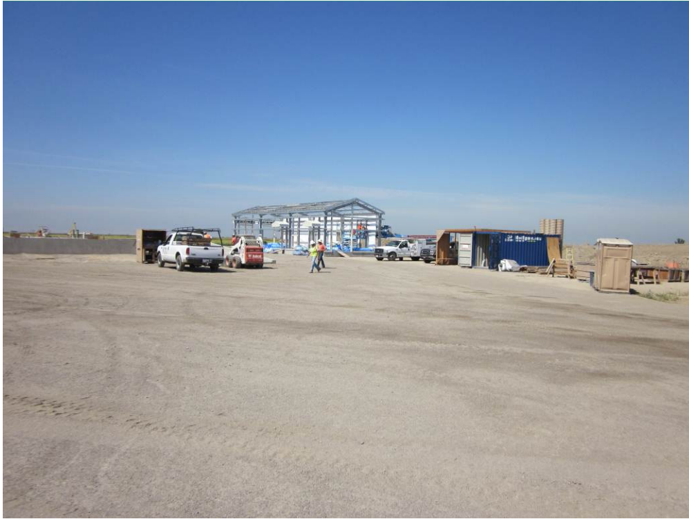
Photo 1: Compressor Station utility building under construction, siding being installed.
