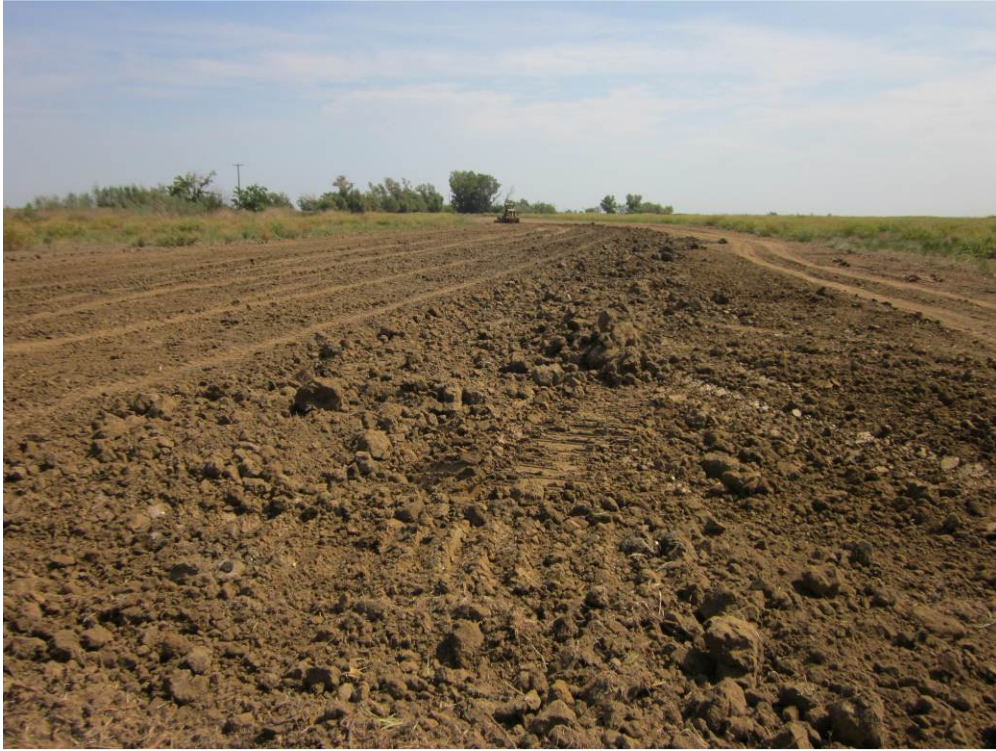
Photo 5: Pipeline right-of-way backfilled, graded and raked east of D-44.
