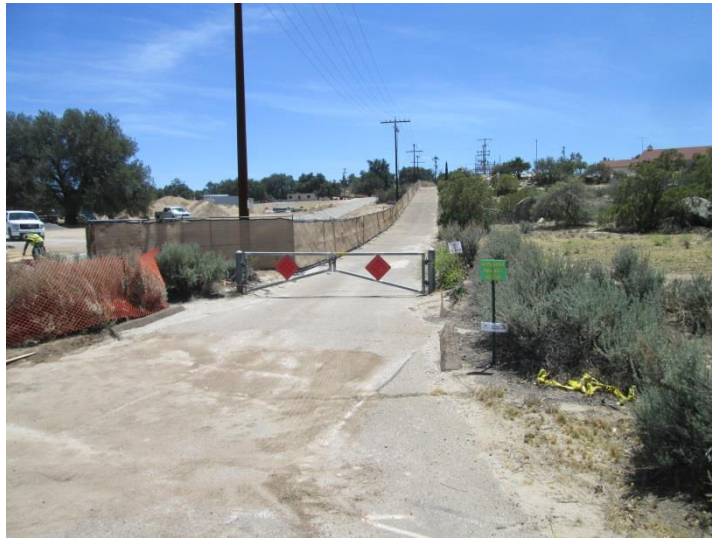
Photo 8: Opaque visual screen fencing was observed being routinely maintained at the Boulevard Rebuild Substation in accordance with MM-VIS-3c.
