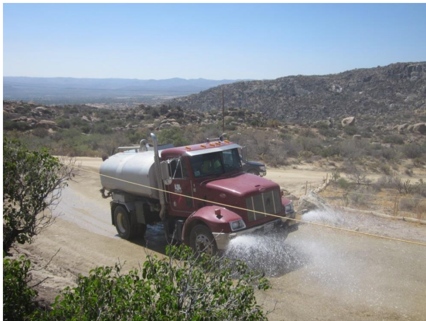
Photo 2: Water trucks being utilized to minimize fugitive dust emissions in accordance with the Dust Control Plan and MM-BIO-4a.
