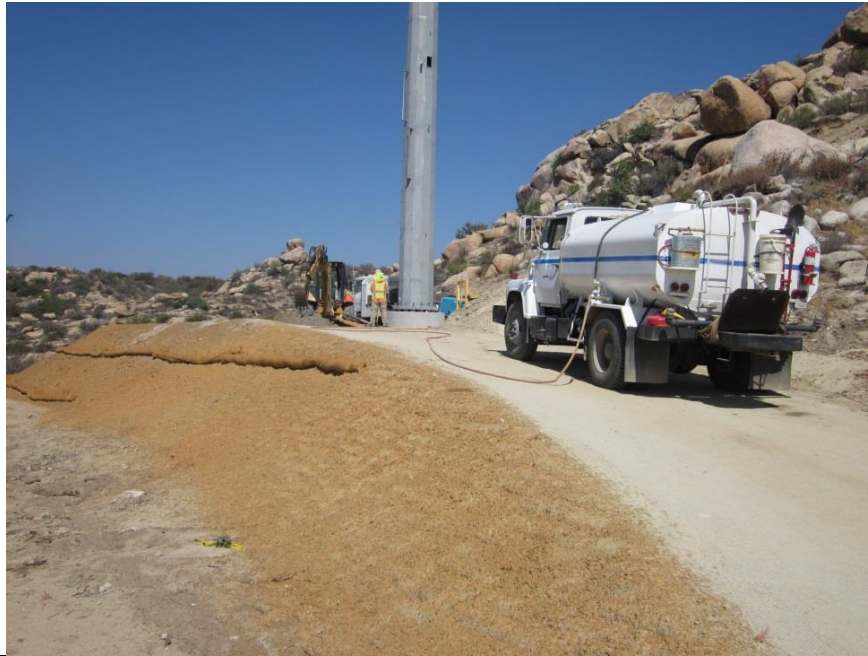
Photo 3: Erosion and sediment controls included the use of straw wattles along the work area perimeter and hydro-mulch on graded slopes (MM HYD-1), and fire tools and water supply were observed on site (FF-1).
