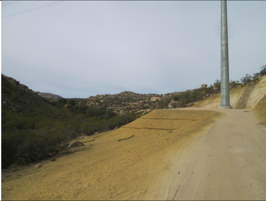
Photo 3: In accordance with MM-BIO-1D and the Habitat Restoration Plan, temporary work areas are stabilized and a seed mix will be applied in the near future. Monitoring to meet the success criteria is required to be completed as described in Section 6.0 of the Habitat Restoration Plan.
