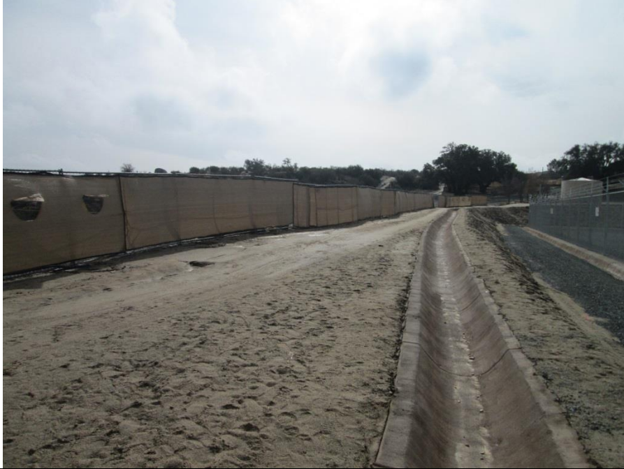
Photo 5: In accordance with MM-VIS-3A, temporary fences along the perimeter of the Boulevard Substation Rebuild are lined with screening material to reduce visibility of construction activities for motorists passing along Old Highway 80.
