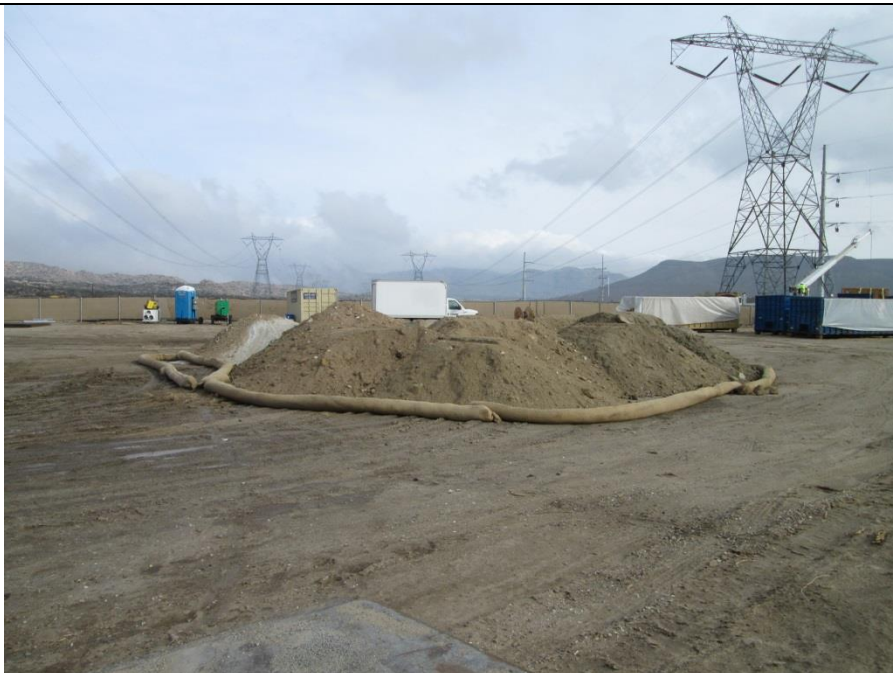
Photo 4: In accordance with MM-HYD-1, straw wattles are placed along the perimeter of spoil piles staged onsite to minimize the potential for erosion.
