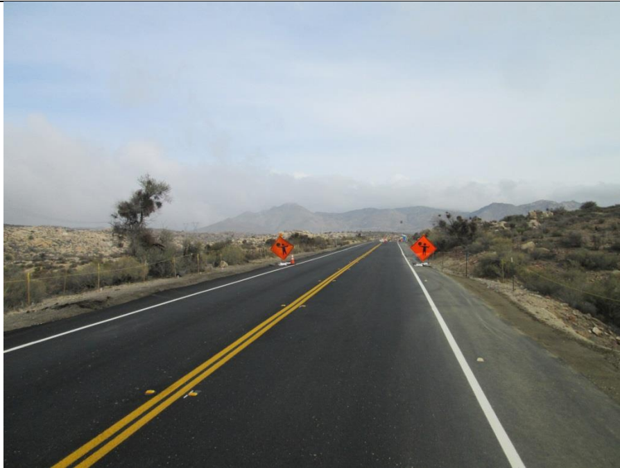
Photo 1: Traffic control measures consisting of signage was observed being implemented along Old Highway 80 in accordance with MM-TRA-1.
