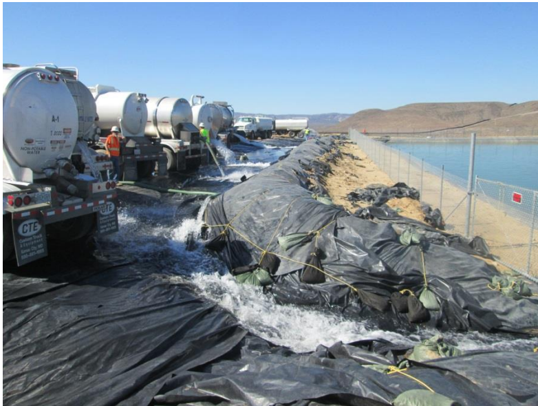
Photo 6: Water trucks deliver water from offsite resources including the City of San Diego, Campo Indian Reservation and Jacumba Community Services District in accordance with MM-HYD-3 and the Amended Construction Water Supply Plan.
