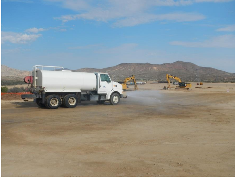
Photo 5: Water trucks are utilized on a regular basis to minimize fugitive dust emissions in accordance with MM-BIO-4A and the Dust Control Plan.
