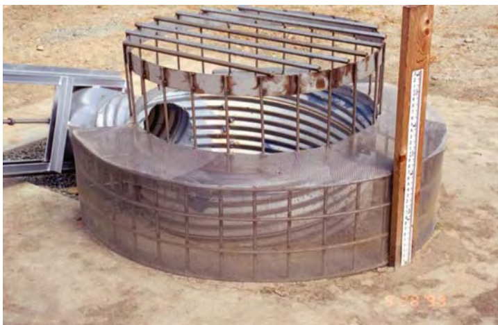
Figure 1 Example of Extended Detention Outlet Structure
